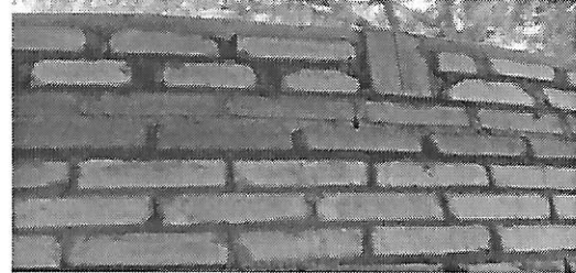
Plate XXXVII: Special (frog) bricks for window lintel, tie beam and roof anchorage.
