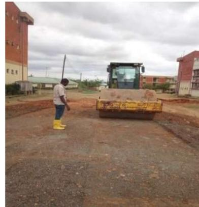
Fig. 8: Field compaction in progress
