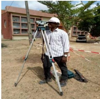
Fig. 6: Theodolite for leveling of subgrade
