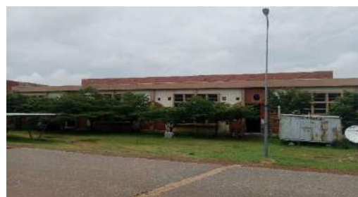
Figure 2: Building main facade and surroundings
