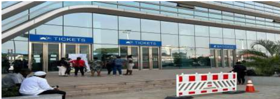
Exterior façade of Mobolaji Johnson Railway Station with glass curtain wall design
