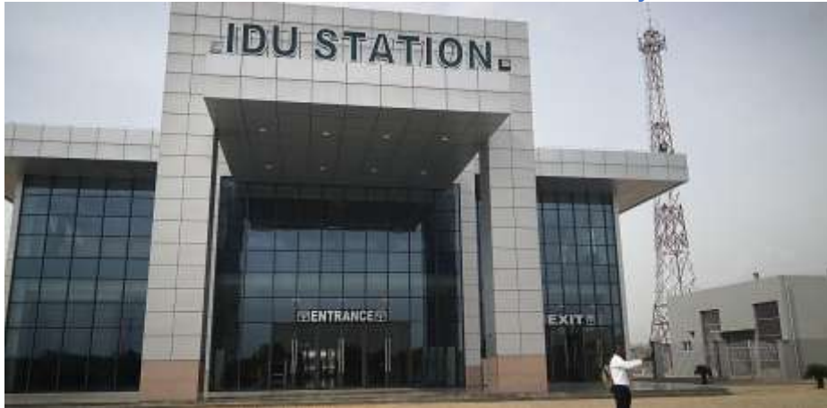
Exterior façade of Idu Railway Station featuring glass curtain walls and metallic cladding
