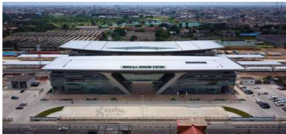
Aerial view of Mobolaji Johnson Railway Station showing Ebute Metta location and urban context
