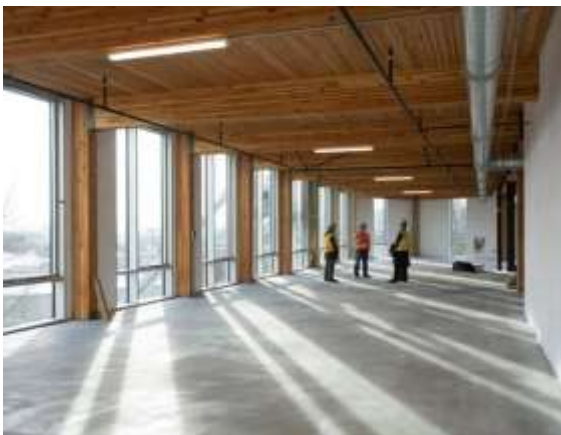
Plate I: Interior of Bullitt Centre, showing the wooden ceiling Source: John Stamets (2013)
