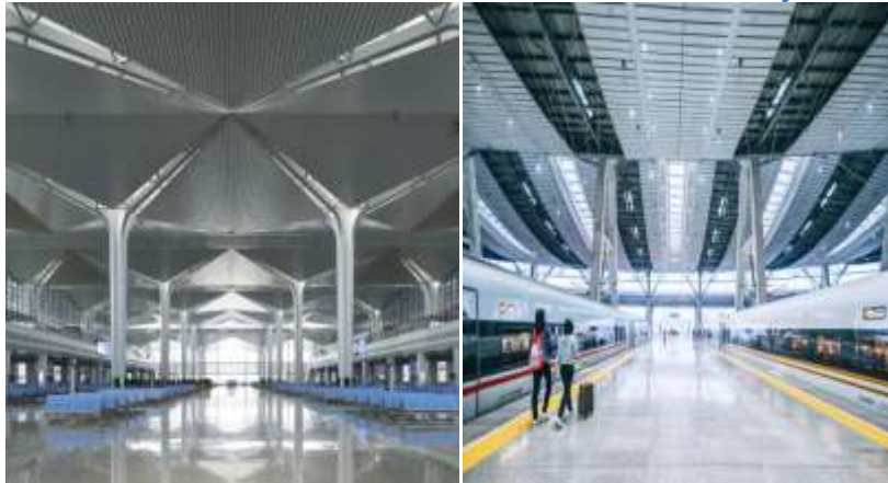
Interior view of Taiyuan South Railway Station showcasing Tang-style Shanxi architecture Source: Jidipi Architectures (2016)
