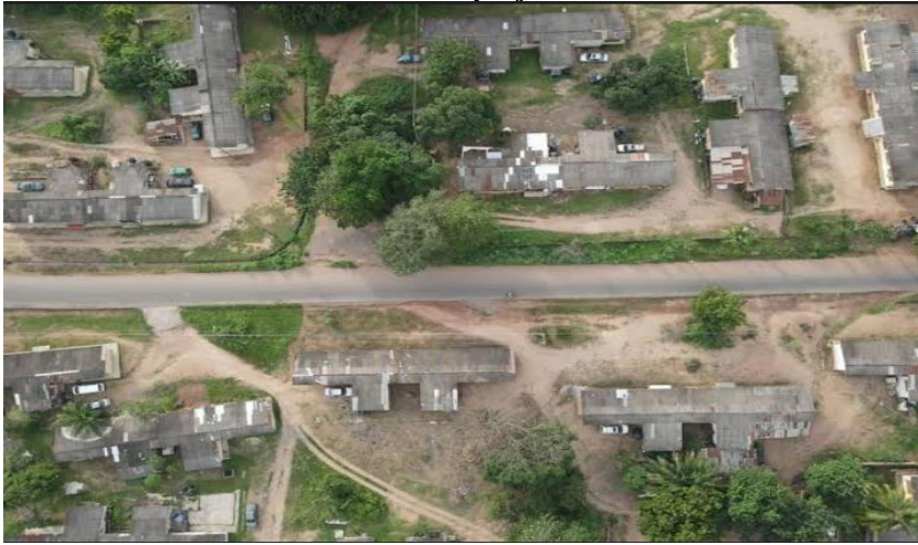
Picture 1: Before the initiation of the project
