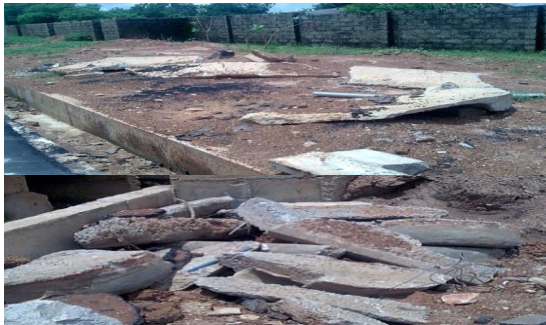
Plate 4: Dutsen kura road concrete waste
