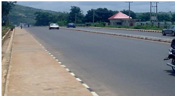
Plate 1: Government House Road
