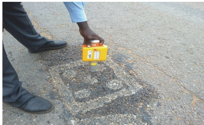
Figure 3: Rebound hammer test
