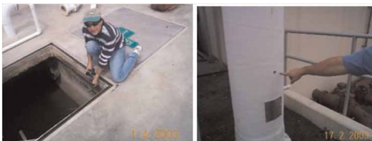
Figure 6. Readings taken in Septage tank (with TRIO 3 permitted authorization).
