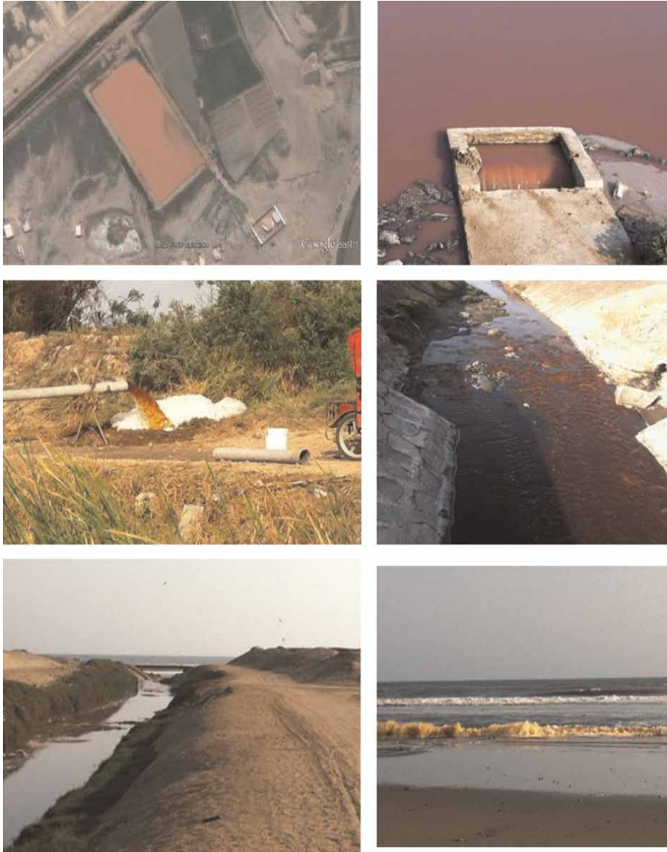
Figure 18. Oxidation lagoon and disposal of treated water in the district municipality of Santa Rosa Lambayeque, Peru (copyright of Reingeniería en Saneamiento ltd).
