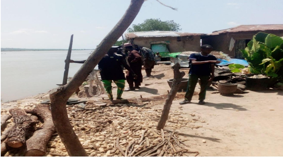
Plate 2: showing the vulnerability of the settlement and some houses in Tsogi community
