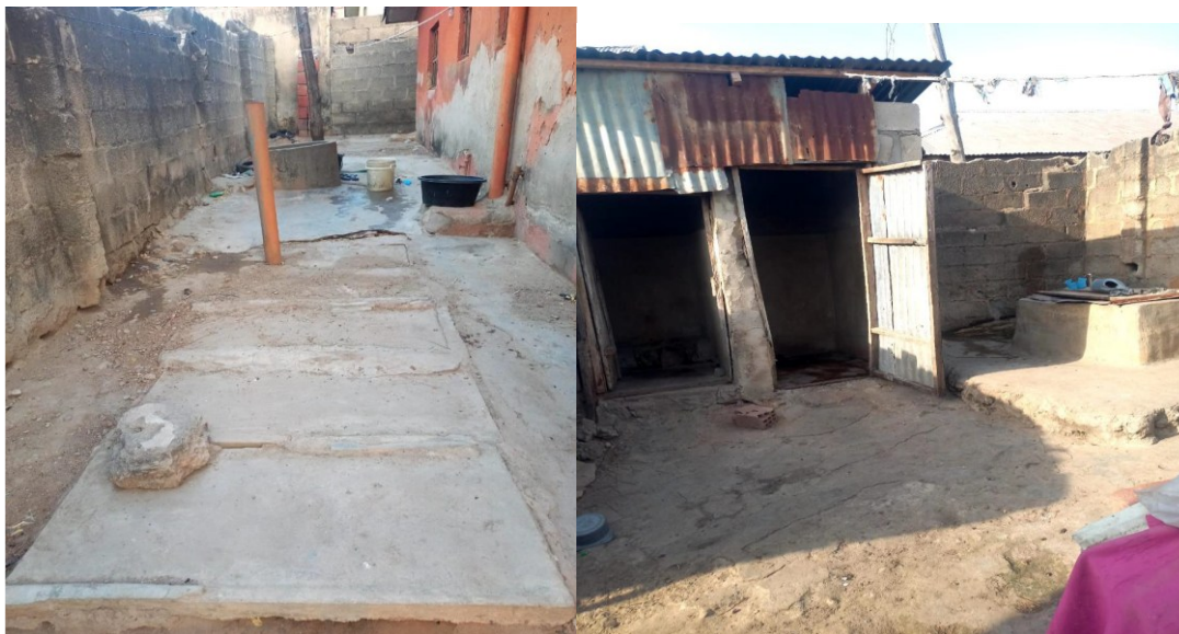
Plate I: Septic Tank around Old Custom Plate II: Toilets Close to Well in Tunga
