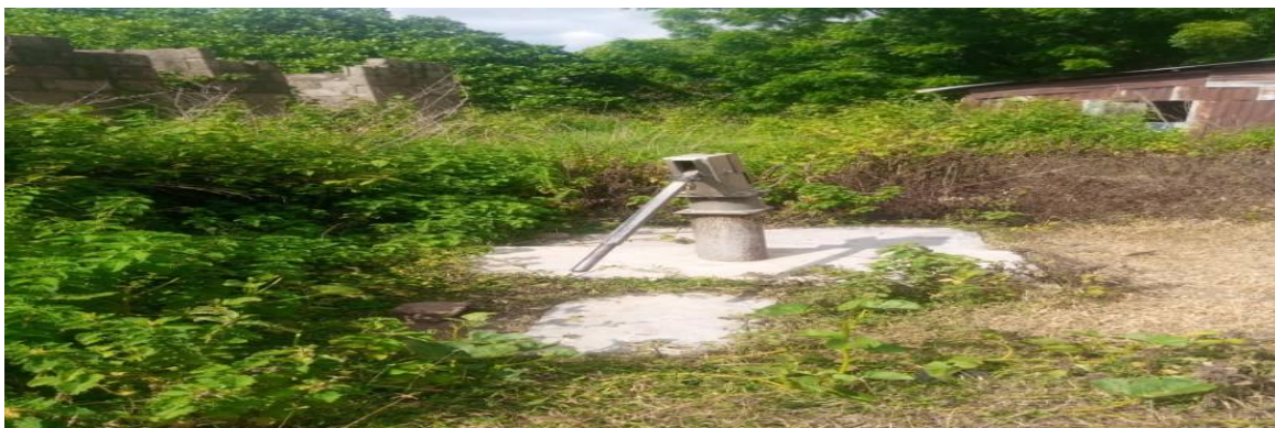
Plate 16: A non-functioning and unsustainable hand pump borehole at Pepelecommunity (MarafaOja) (PHP2)
