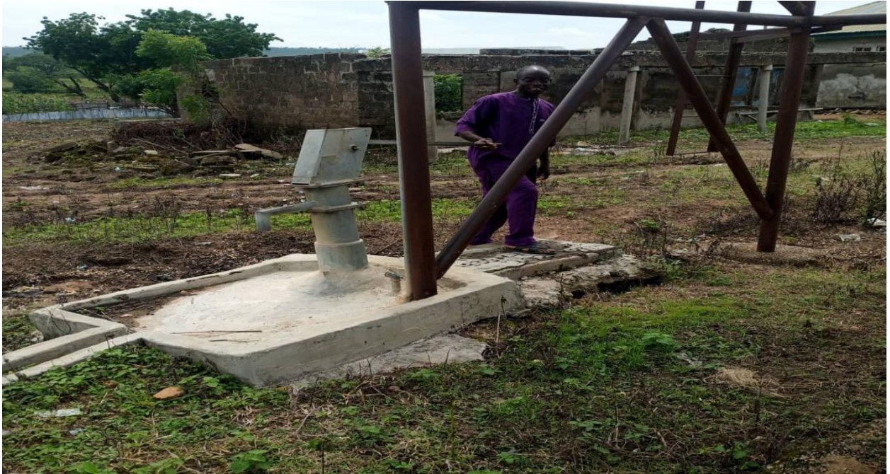
Plate 11: A non-functioning and unsustainable hand pump borehole at Apado community (AHP7)
