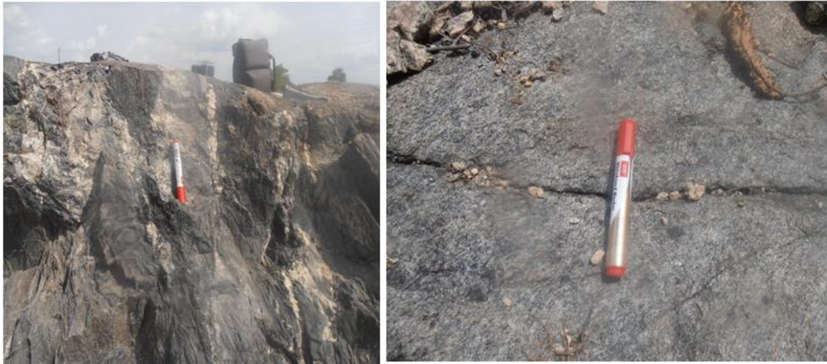
Fig .11. Joints fractures and fault were other structure attribute found among the basement rocks in the study area
