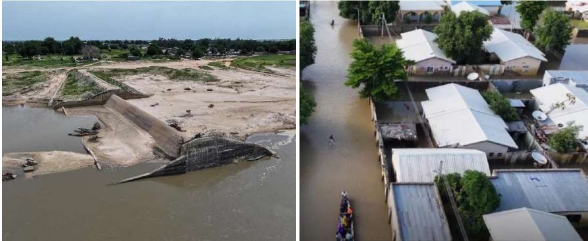
Figure 4: The concrete spillway and crest of the Alau dam and the flooding after the dam collapsed in northeastern Nigeria. (Source: New York Times of Oct. 27, 2024; Photographs by Fati Abubakar Ruth Maclean, Ismail Alfa and Fati Abubakar reported in New York Times of Oct. 27, 2024)
