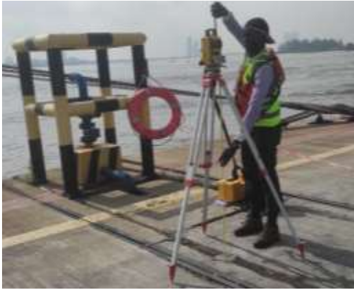
Figure 5(a) Setting up the Total station
