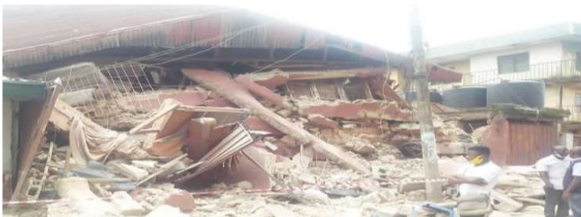
Plate 3 shows a recent reported case of Collapsed Buildings in Jos Metropolis, plateau State
