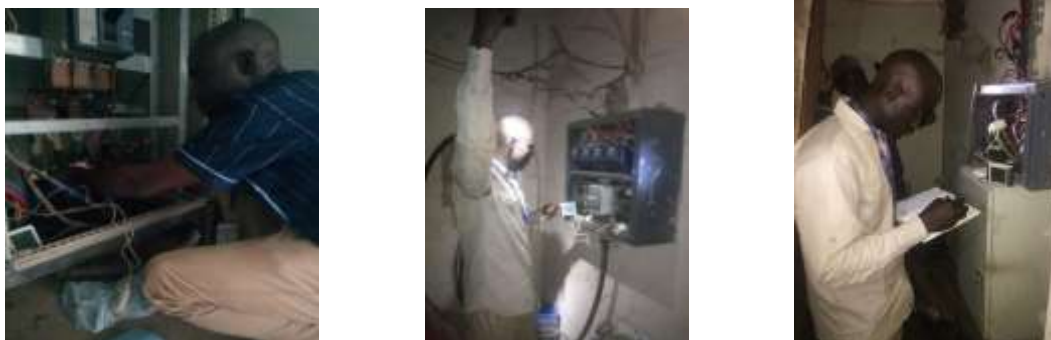
Figure 3.2: Clipping the jack-plug on the live wires at Zungeru Polytechnic and Niger State College of Education administrative blocks the main panel distribution board (MPDB).
