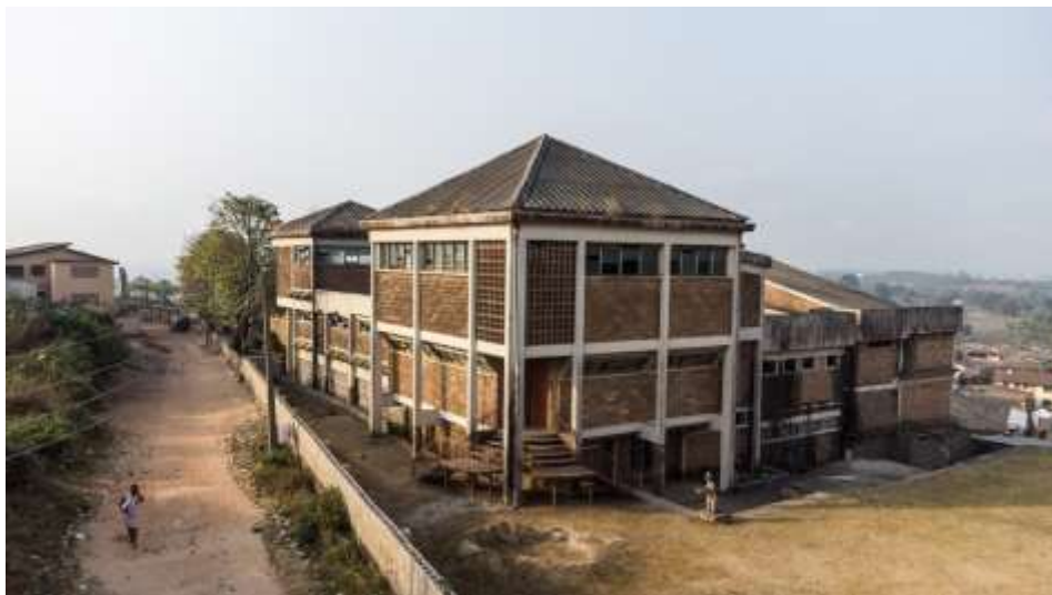
Figure 6: Approach view of the Cultural Centre Ibadan.
