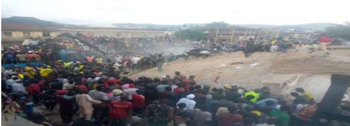
Plate 1 shows Scene of a collapsed building in Jos by James Abraham (3rd October 2020)
