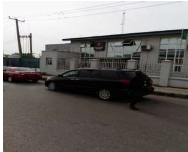
Plate II: Parking Facilities at Polaris Bank II, Old Airport
