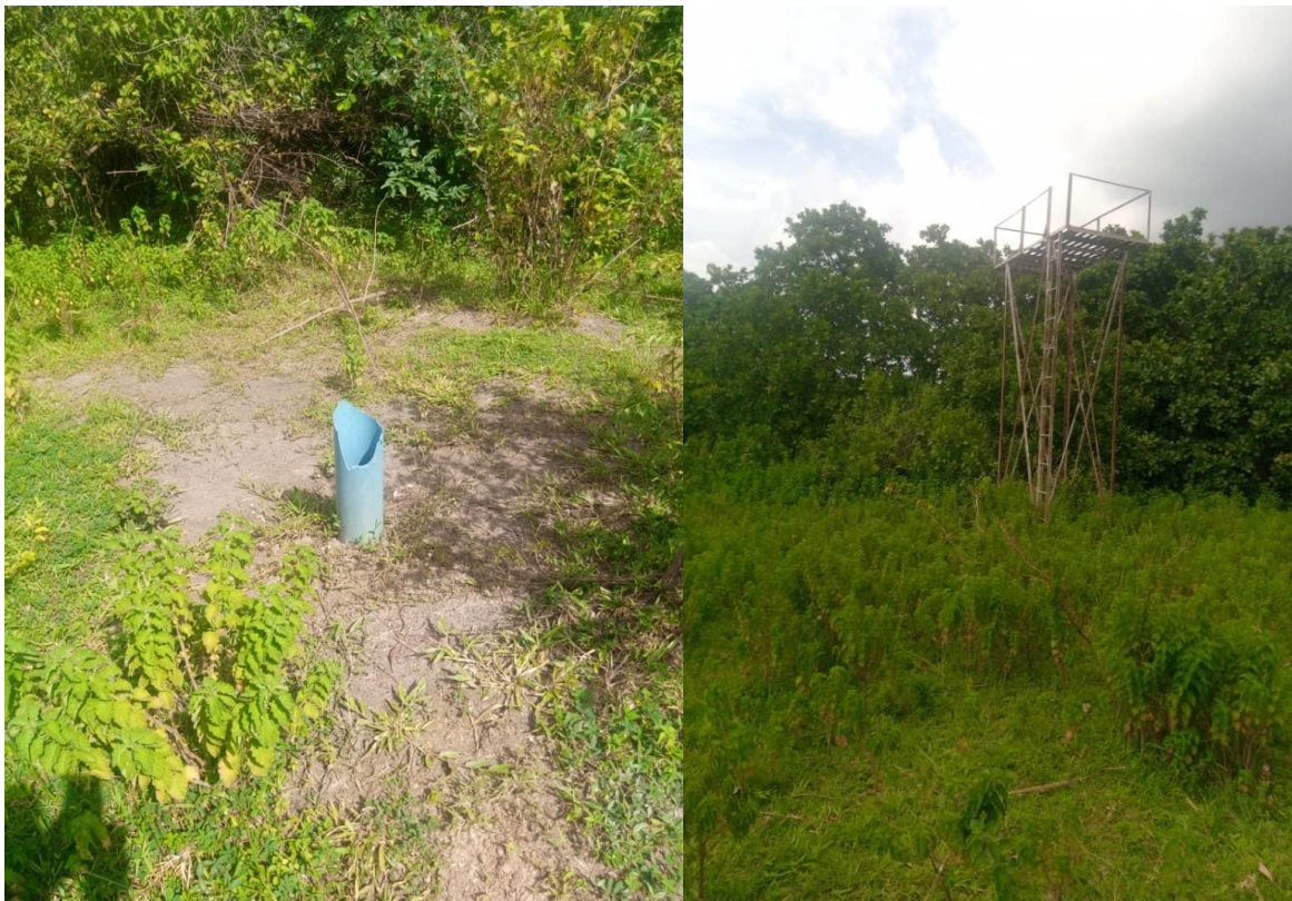
Plate 13: A non-functioning and unsustainable motorized borehole at Pepelecommunity(MarafaOja)(PMR3)
