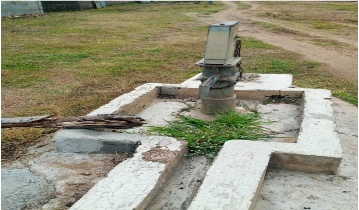
Plate 9: A non-functioning and unsustainable motorized borehole at Apado community (AHP5)
