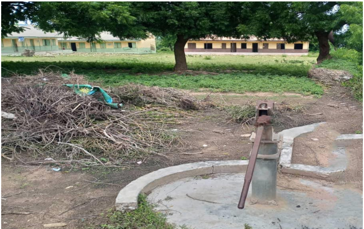
Plate 10: A non-functioning and unsustainable hand pump borehole at Apado community (AHP6)
