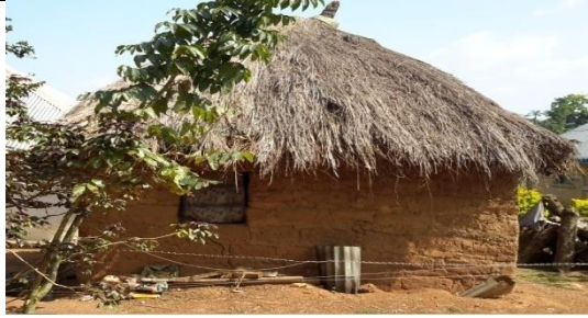
Plate VIII: Traditional housing made with mud wall and thatch grass roof
