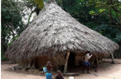
Plate X: Traditional housing made with mud wall and thatch grass roof.
