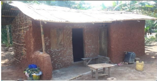
Plate VI: Wattle and daub construction of traditional housing made with mud wall and transformed zinc roof.
