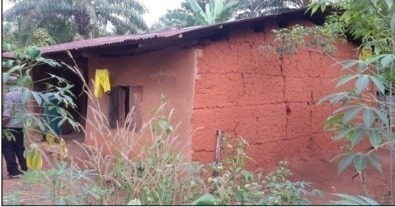
Plate IV: Traditional Residential House of Late Mr. Ikebuaso Ofolagoro of Ihite-oha Orsumoghu, Ihiala L. G. A, Anambra State. Showing Transformation on Roof and Plaster on the Mud wall.
