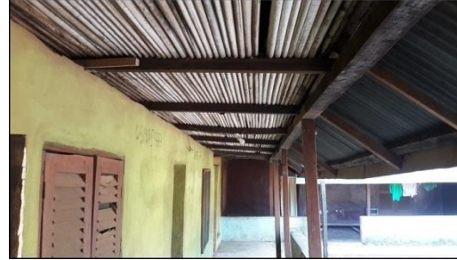
Plate V: Late Mr. Humphrey Okuma's Transformed Traditional Building at Ihiala built in 1960, showing timber post, raffia palm ceiling, mud wall plastered with cement and roof covered with zinc.
