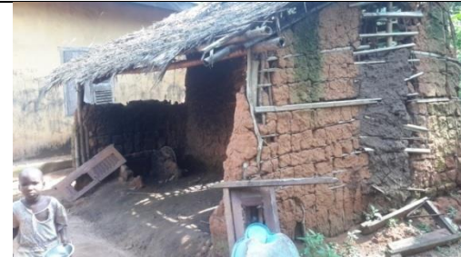
Plate VII: Wattle and daub construction of traditional housing made with mud wall and thatch raffia palm leaves roof.
