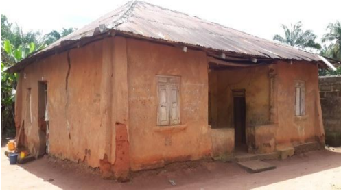
Plate XII: Transformed traditional housing made with laterite wall, plastered with cement plaster and covered zinc roof.
