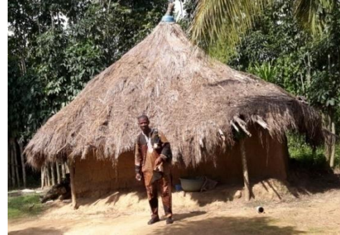
Plate XI: Researcher posing at the traditional housing made with mud wall and thatch grass roof.
