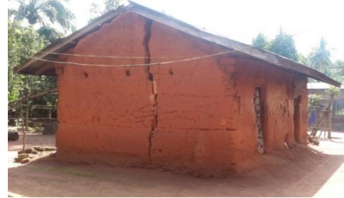
Plate XIII: Transformed traditional housing made with laterite wall, and covered with zinc roof.
