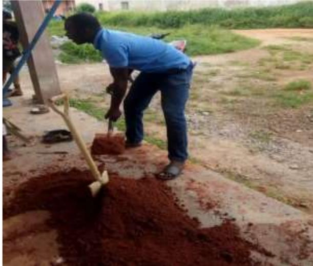
**Plate VI Mixing of the laterite with the additive**
