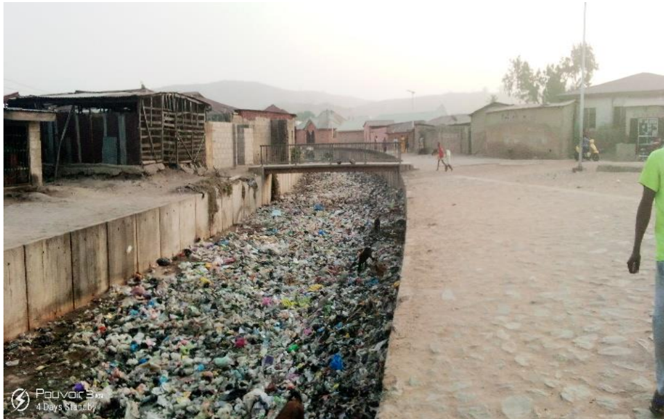
Plate 1: Blocked Barger drainage in Minna-West Central
