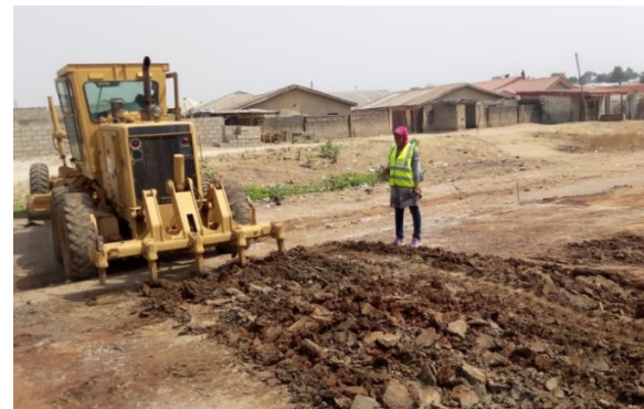
Fig. 2: Scarification of the test sections using ripper
