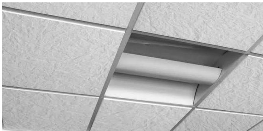
Figure 2.10. Suspended ceiling made with mineral fibre
