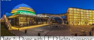
Plate 7: Dome with LED lights (conserve energy) LOCATED IN A VERY ACTIVE EARTHQUAKE REGION, THE STEEL STRUCTURE WAS BUILT AS A WELDED TRIANGULAR SPACE FRAME WHILE THE HOTEL AND THE OFFICE BUILDINGS HAVE BEEN DESIGNED AS SKELETON STRUCTURE OF REINFORCED CONCRETE FEATURING HIGH FLEXIBILITY.
