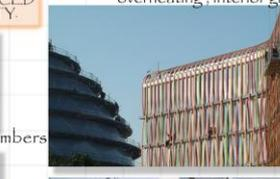
Plate 11: External wood cladding shielding fenestrations with green loggias serving as buffer zone, cooling the air thereby creating a pleasant indoor climate
