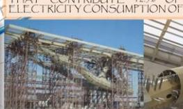
Plate 13: Roof deck and steel structure of the tree-shaped organic metal columns
