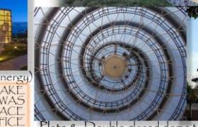
Plate 8: Double glazed dome to prevent the interior from overheating, interior glass was created using lamellae
