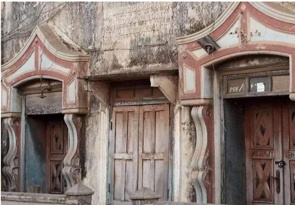
**Plate XI: Cornice design around doors and windows openings.**
