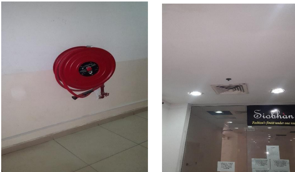
Plate VII: The fire control horse reel and water sprinkler with HVAC.
