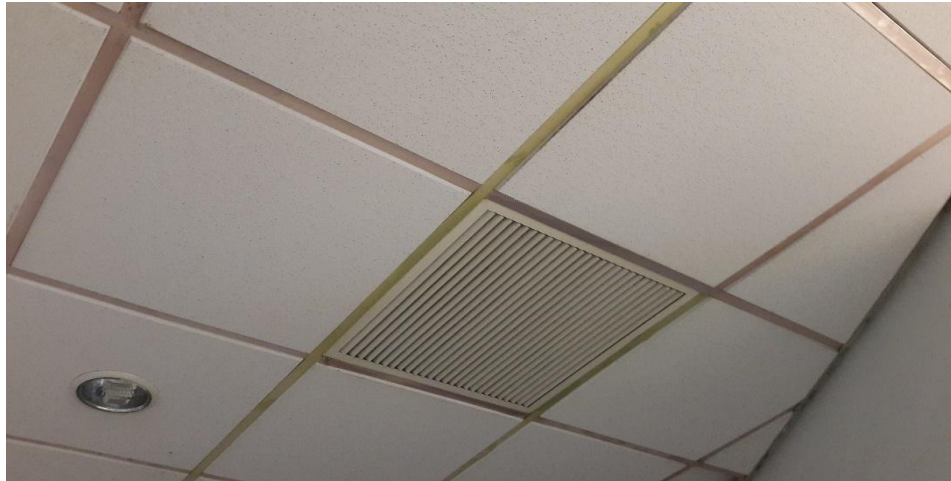
Plate II: Fire-resistant ceiling
