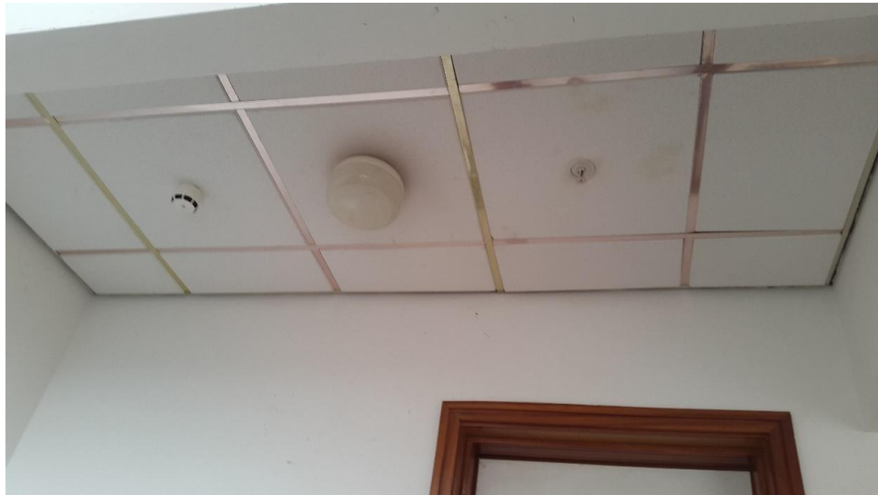
Plate IV: The fire sprinkler and smoke detector.
