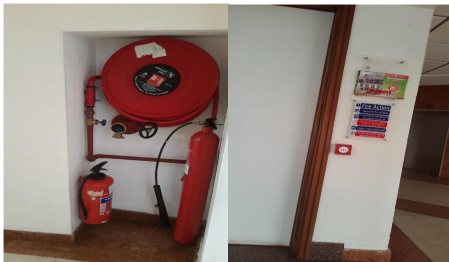
Plate III: The fire horse, extinguisher and alarm button.
