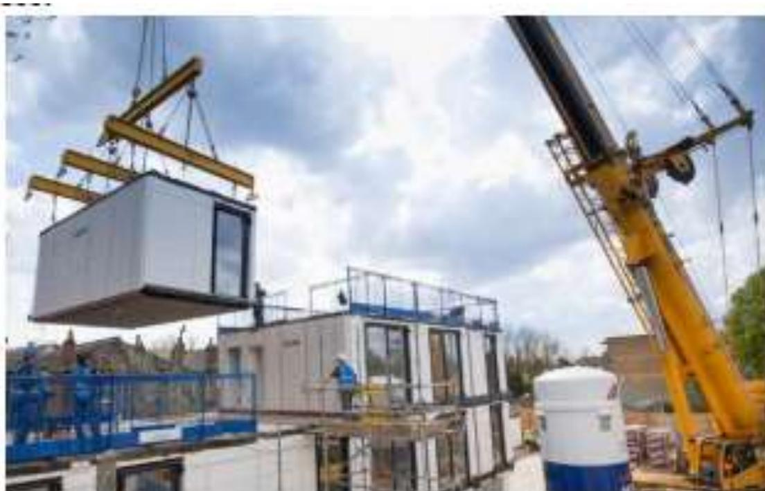
**Figure 2.1: Installation of Modular Home**
