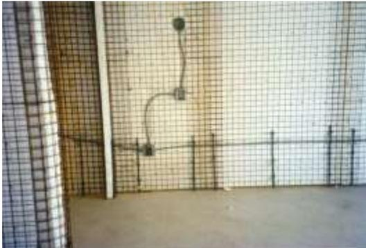
An EPS wall erected with conduit pipes fixed in it.
