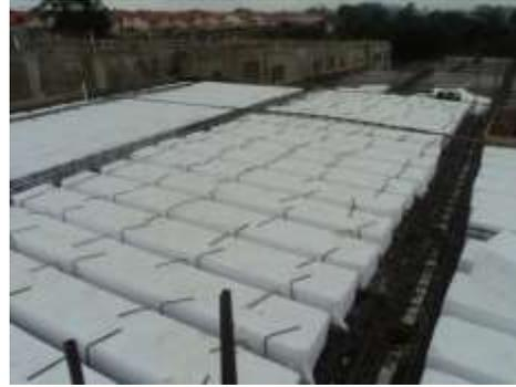
Reinforcement being fixed for an EPS slab
