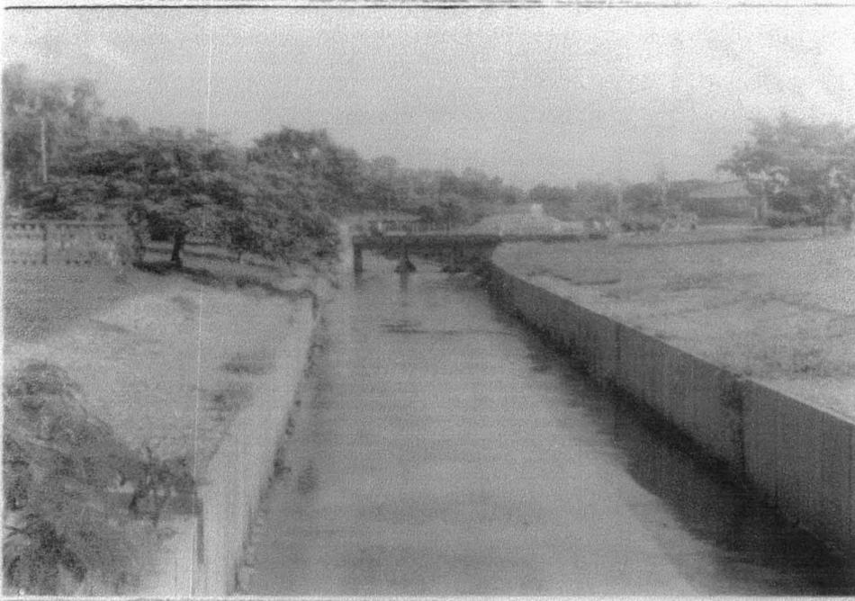
Plate 1: The drainage channel that cut across the Bosso campus of F.U.T, Minna, Was concretized to protect the Bank against collapsing.
