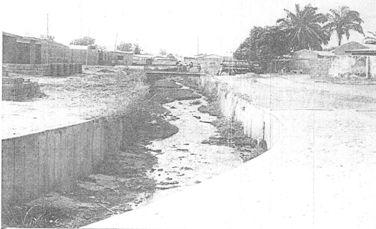
Plate2: Terminal point of the Tunga drainage system. Note the Pillars used as means of reducing the velocity of the water
