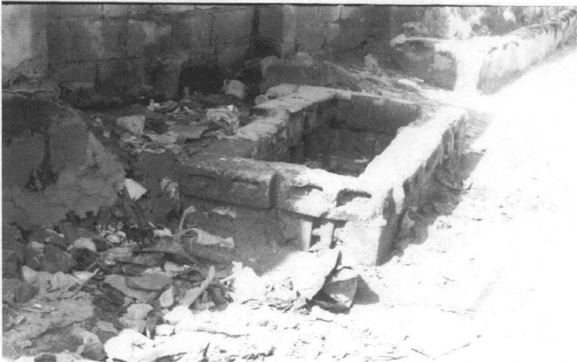
Plate 4.4 This is a picture of soak away pit with waste deposited within its surrounding at Sabon Gari Unguwan Arewa Kontagora.
