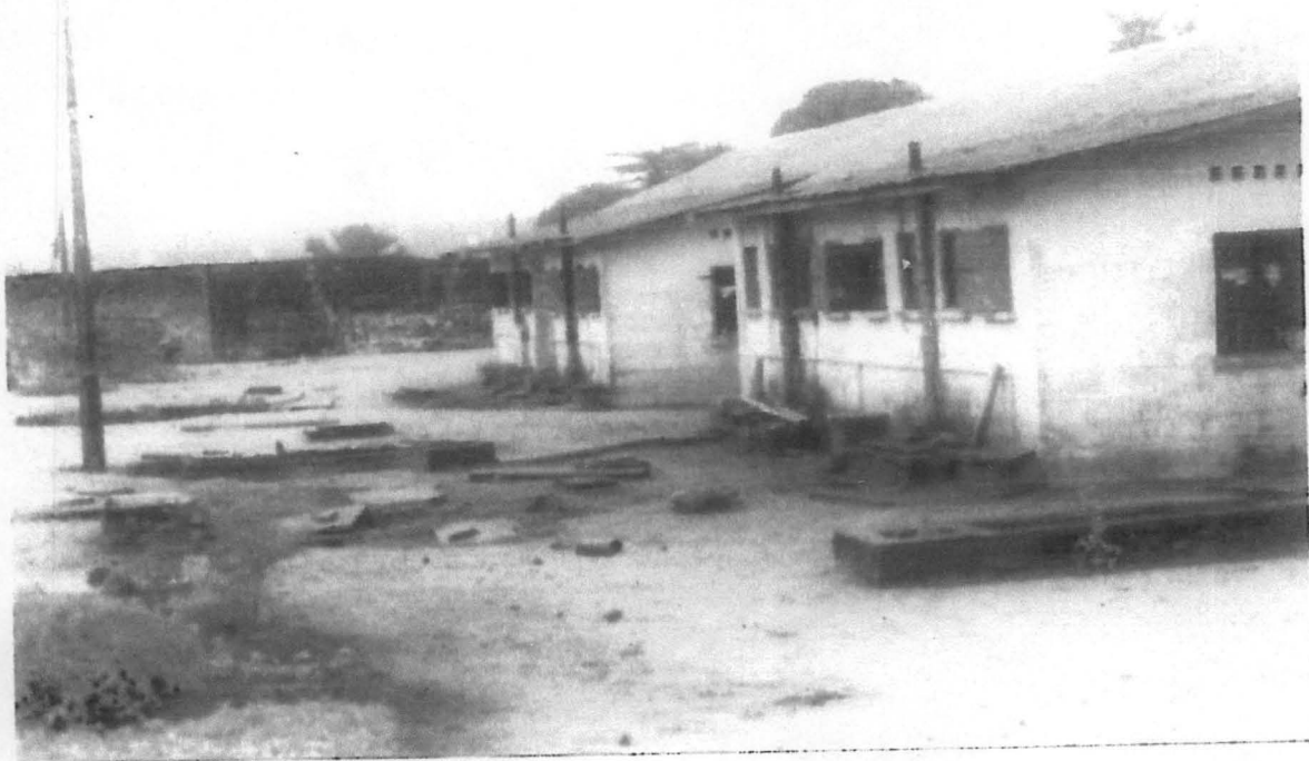
Erosion exposed Prisons structure
