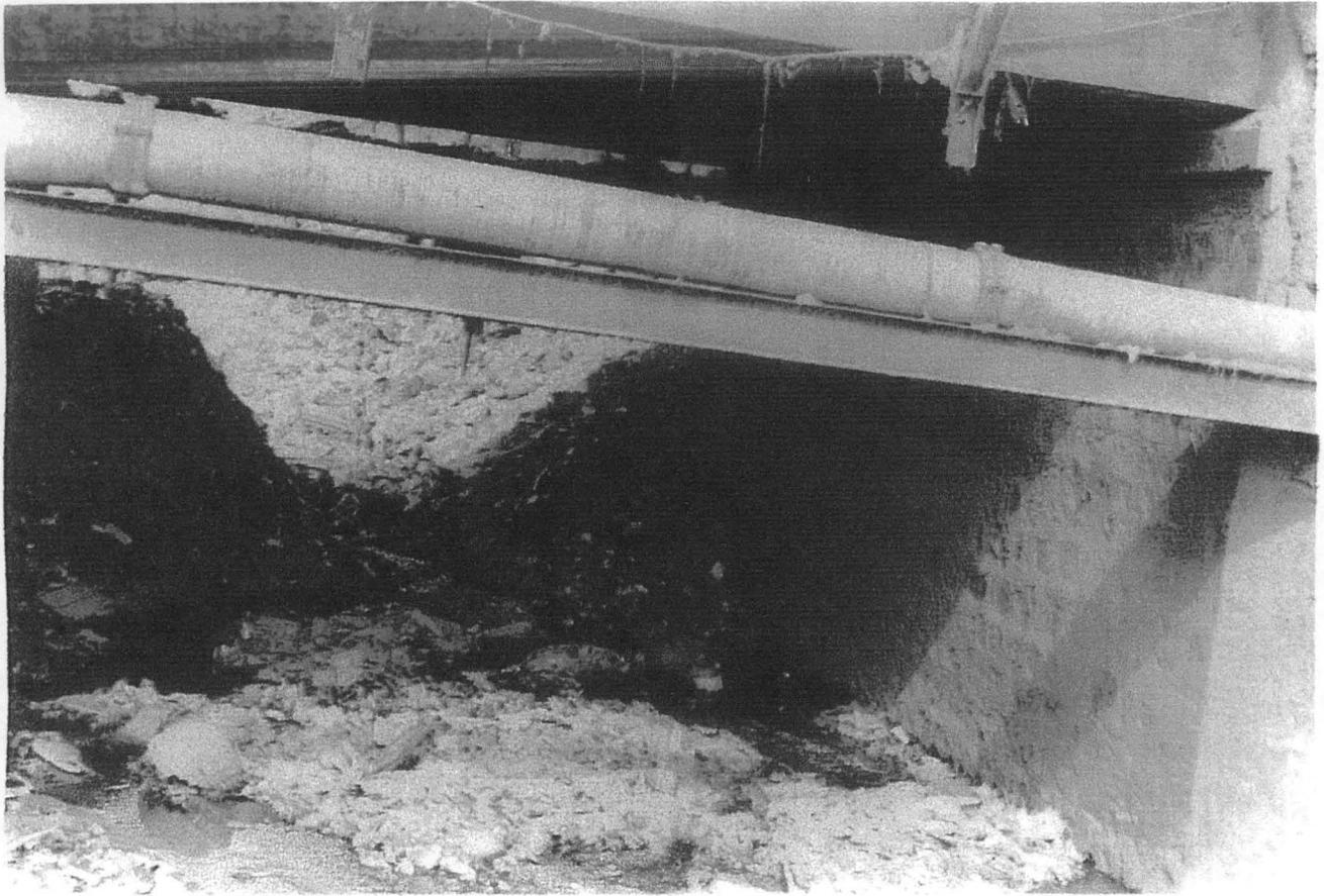
**Plate 7: Refuse blocking a concrete Bridge in Suleja.**
