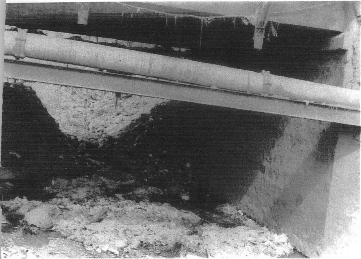
Figure 7: Refuse blocking a concrete Bridge in Suleja.
