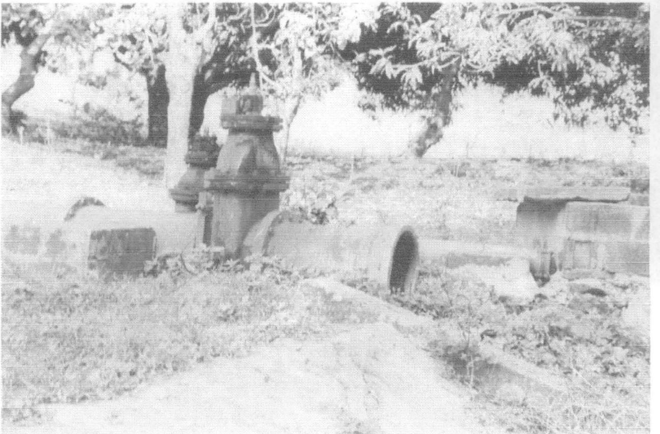
**Plate 13:- Showing vandalized equipments (Pipes) at the reservoir.**
