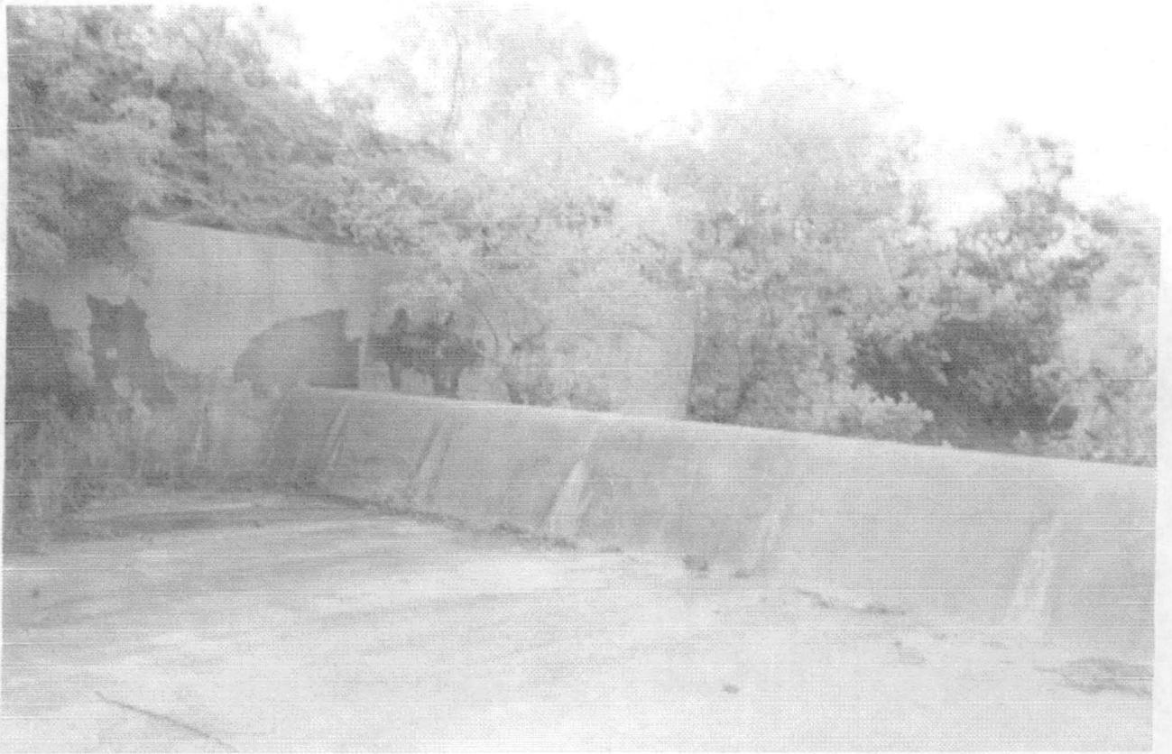
**Plate 12:- Showing Eroded fringes of the reservoir at the Spillway.**
