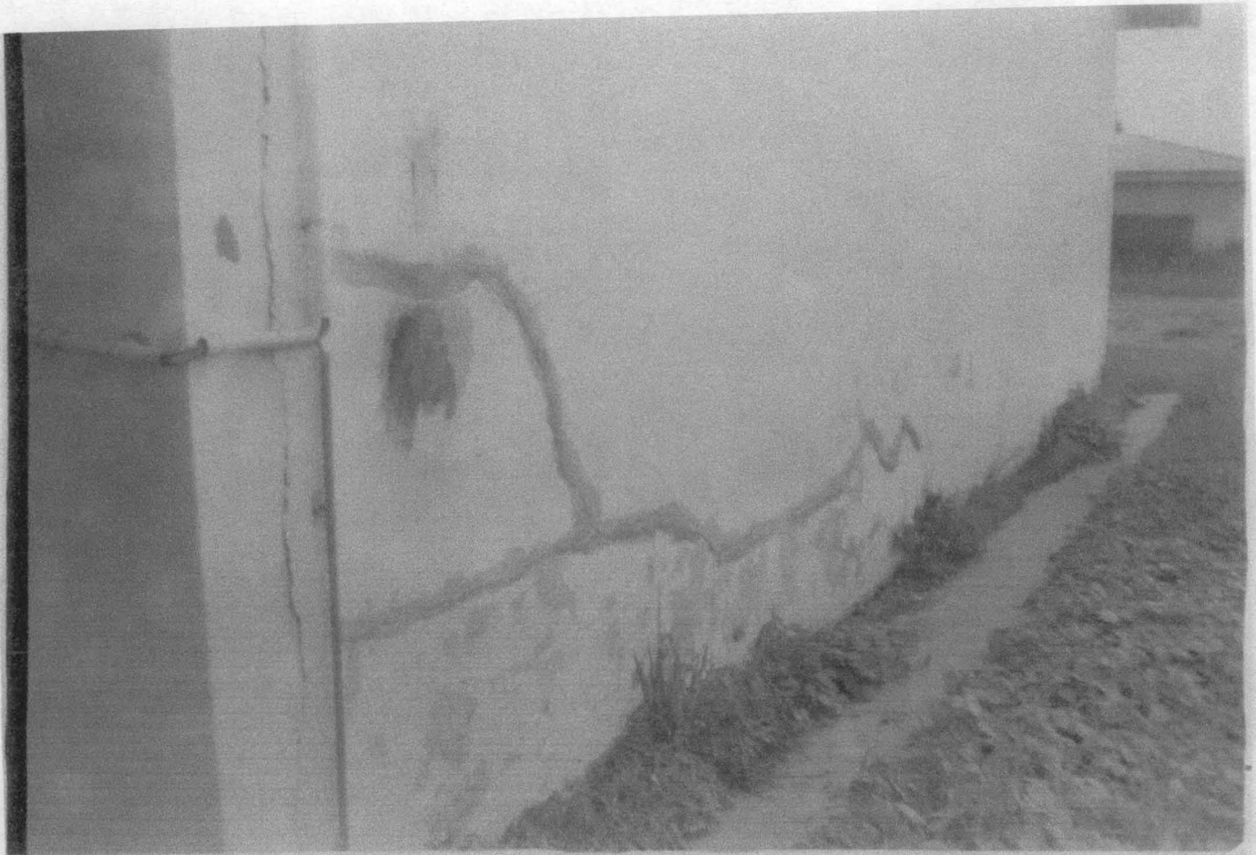
PLATE 3: CRACKED WALL DUE TO VIBRATION FROM BLASTING
