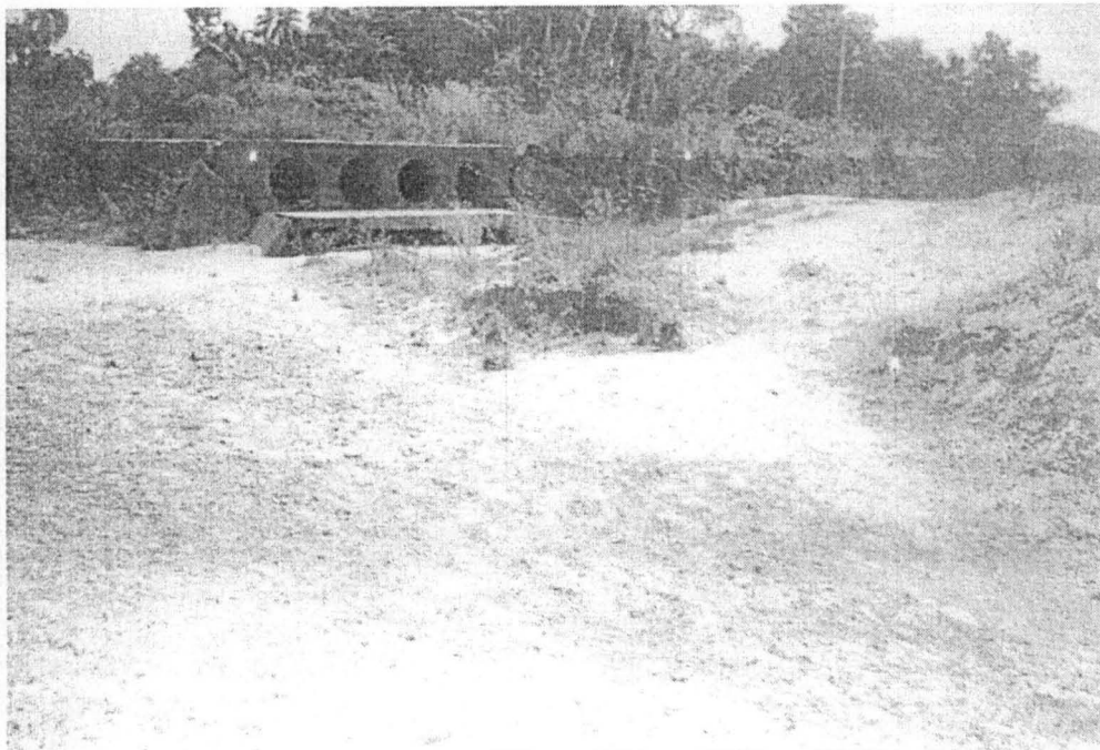
PLATE 4 - Gully erosion along Takpagi Yiba Road. The bridge eroded away – Excessive deforestation long Guineas farm.
