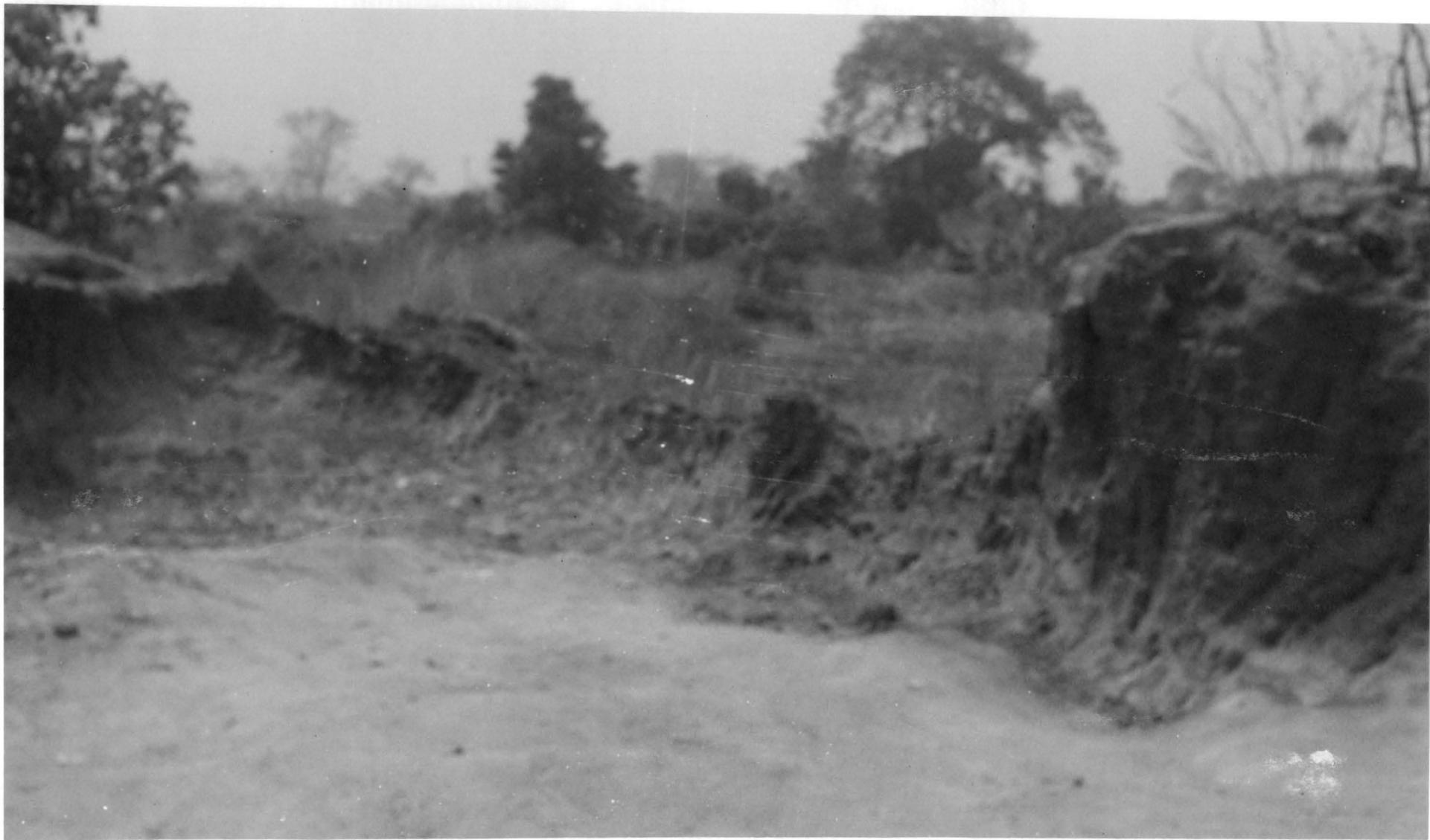
**Plate 10: Showing effect of construction activities resulting in the loss of land to borrow pits/mining of laterite and gravel.**
