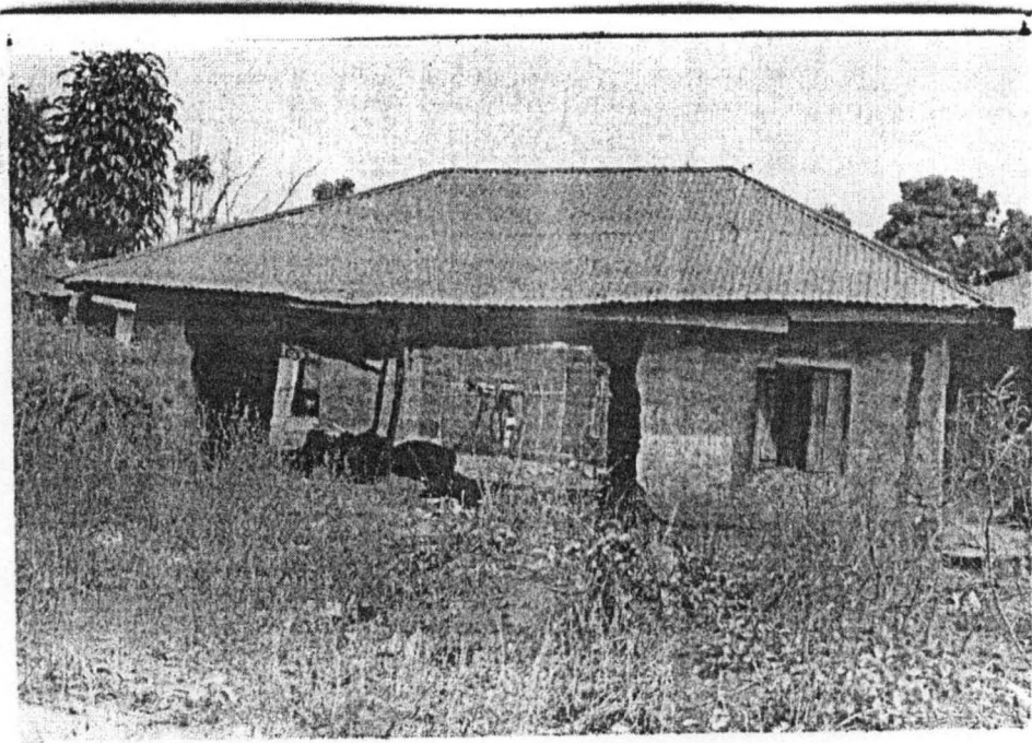
plate 1 Many houses in this area are falling and sticks are used to support the roof while people still living in. (Source: Author's Field Photograph)
