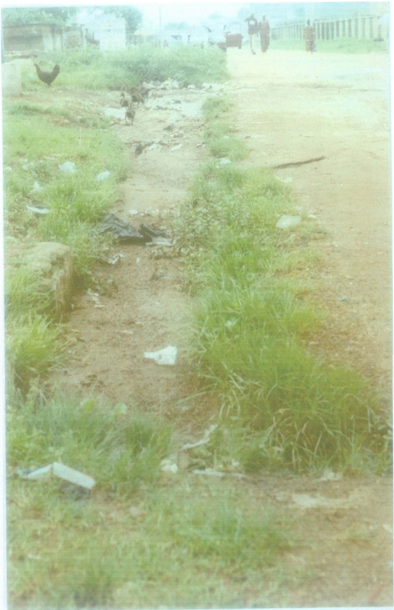
A blocked drainage
