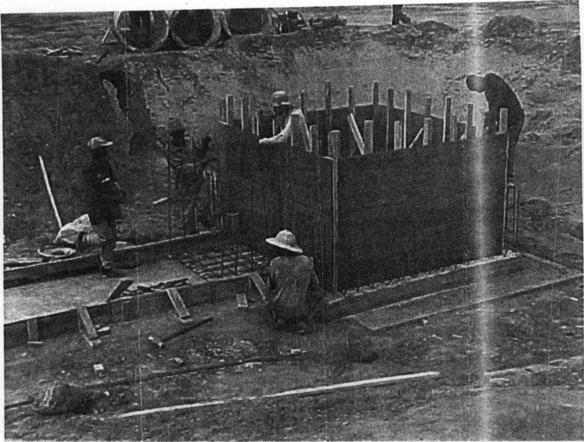
**GROUP A:** MISCELLANEOUS PROTECTION WORK: KETA 900mm DIAMETER RING PIPE CULVERT ; BLINDING, REINFORCEMENT AND FORMWORK FOR THE SUMP.
