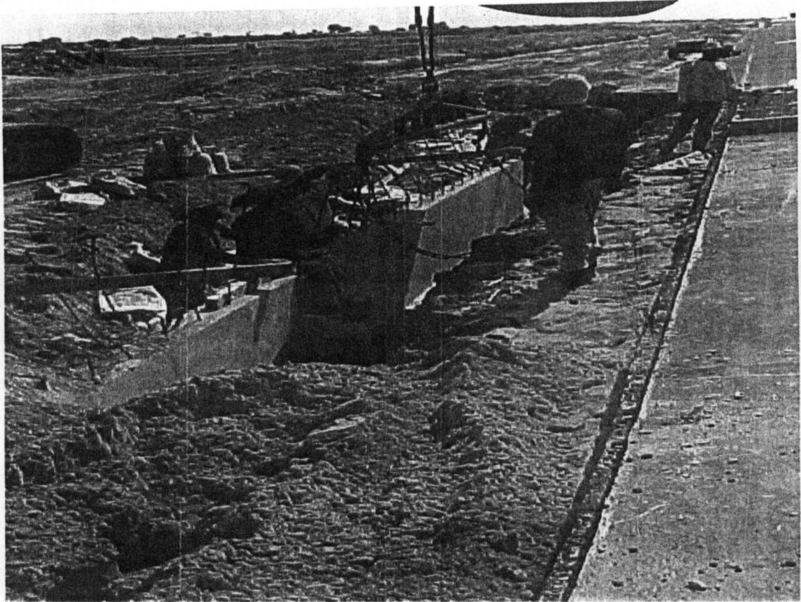
**GROUP T2** : EMERGENCY SPILLWAY; PLACEMENT OF ANCHOR BEAM.
