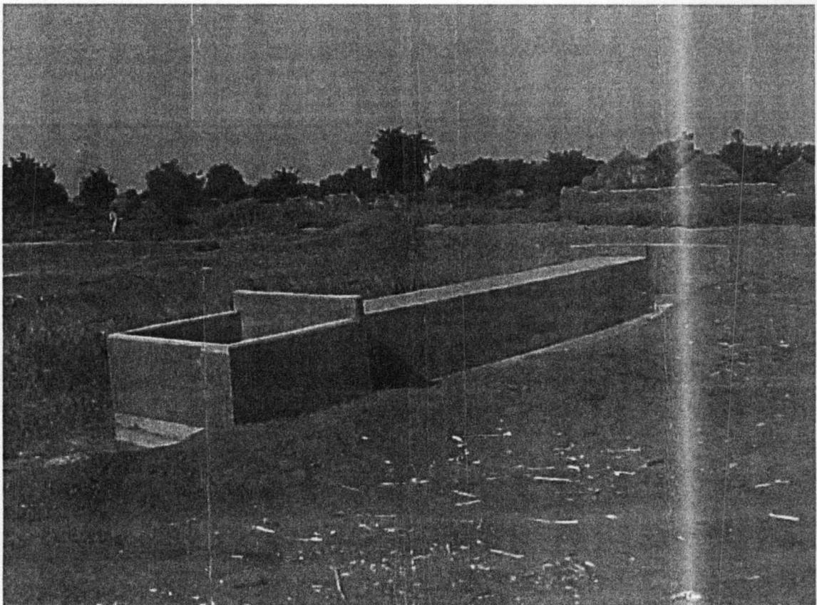
**GROUP B:** MISCELLANEOUS PROTECTION WORK: COMPLETION OF ~~KETA~~ 900mm DIAMETER RING PIPE CULVERT.
