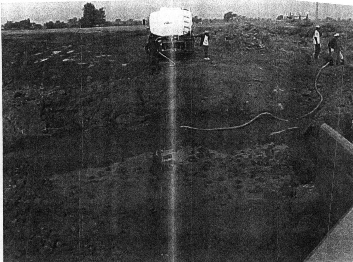
**GROUP G:** MAIN DRAINAGE CANAL NO.1, PLACEMENT OF FILTER BEDDING.
