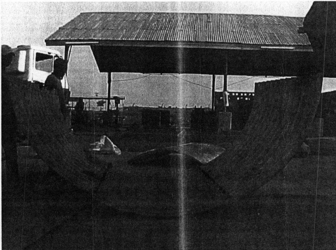
**GROUP 64 :** MAIN DAM STILLING BASIN; PREPARATION OF STEEL PANELS AT YARD FOR DIVERSION CHANNEL.
