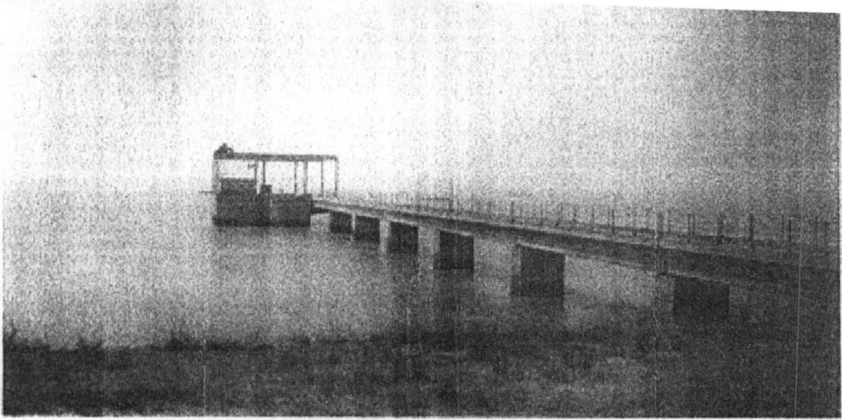
**ATE NO 9: ACCESS BRIDGE LEADING TO THE BULKHEAD GATE CONTROLLING CRANE AND METEOROLOGICAL EQUIPMENT.**
