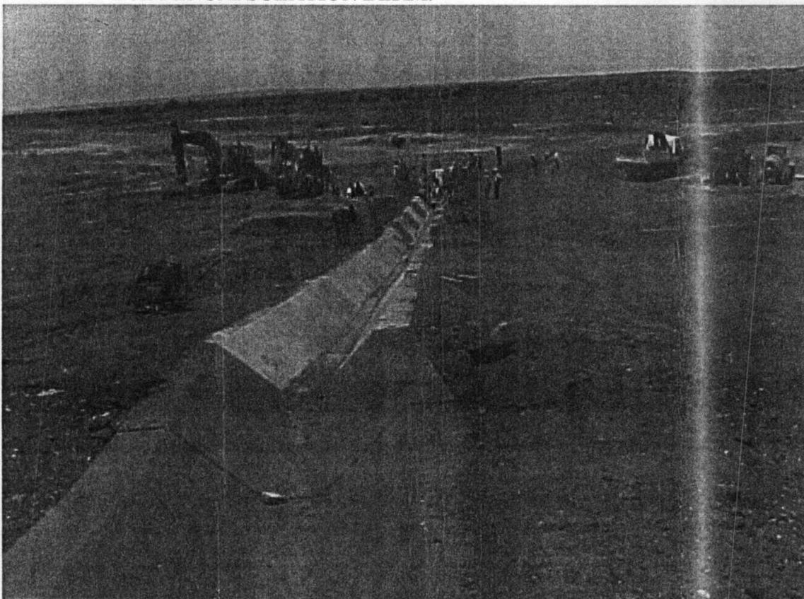
**GROUP P: ROAD SECONDARY- SADDLE DAM ; CONCRETE LINED DRAINAGE CHANNEL TOWARDS INLET OF CULVERT AT CH 0+090.**
