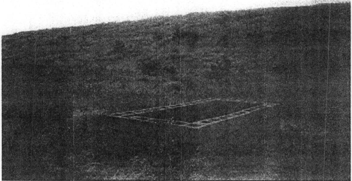
**PLATE NO 5:      RECTANGULAR CONSTRUCTION THROUGH WHICH FLOWS FROM TOE DRAIN ARE MEASURED BY MEANS OF V-NOTCH WEIRS.**
