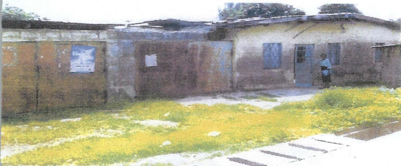
**Plate 1:** The effect of rainstorm on a house; Wind has blown off Part of the roof, discoloured paint surface, corroded metal gate, roofing timber, fascia, board and ceiling board decayed due to moisture.
