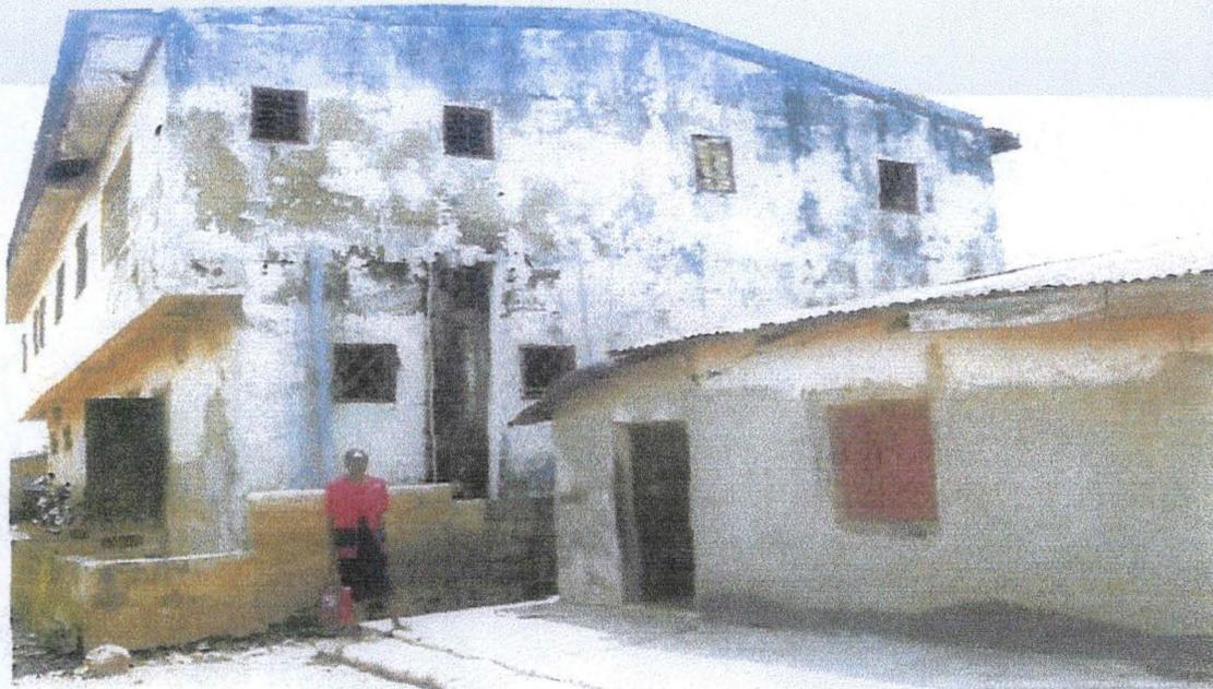
**Plate 9:** Shows the effect of rain on a storey building washing of the paint and damp penetration at the top part of wall surface.
