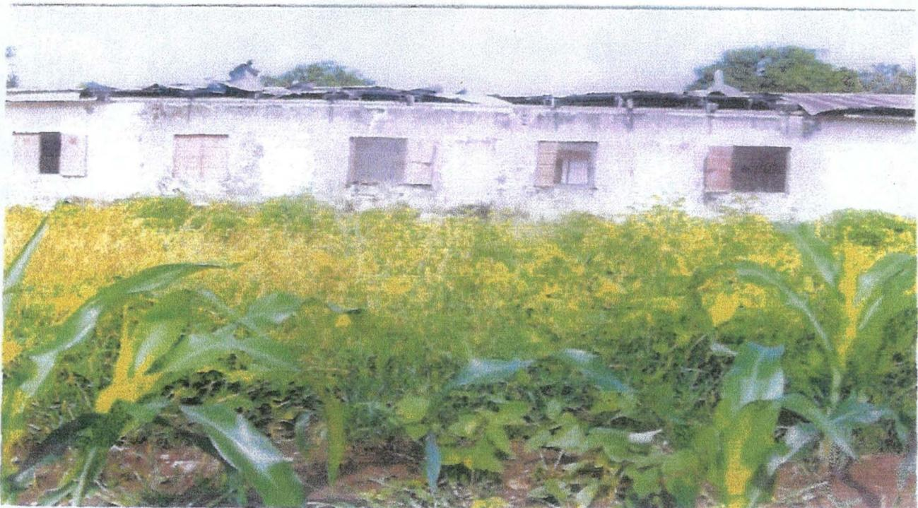
**Plate 6:** The effect of rain washing away the paint on wall and Wind blowing off part of the roofing sheet. Also part of Fascia board and ceiling board completely falling off in G.T.C. Minna.
