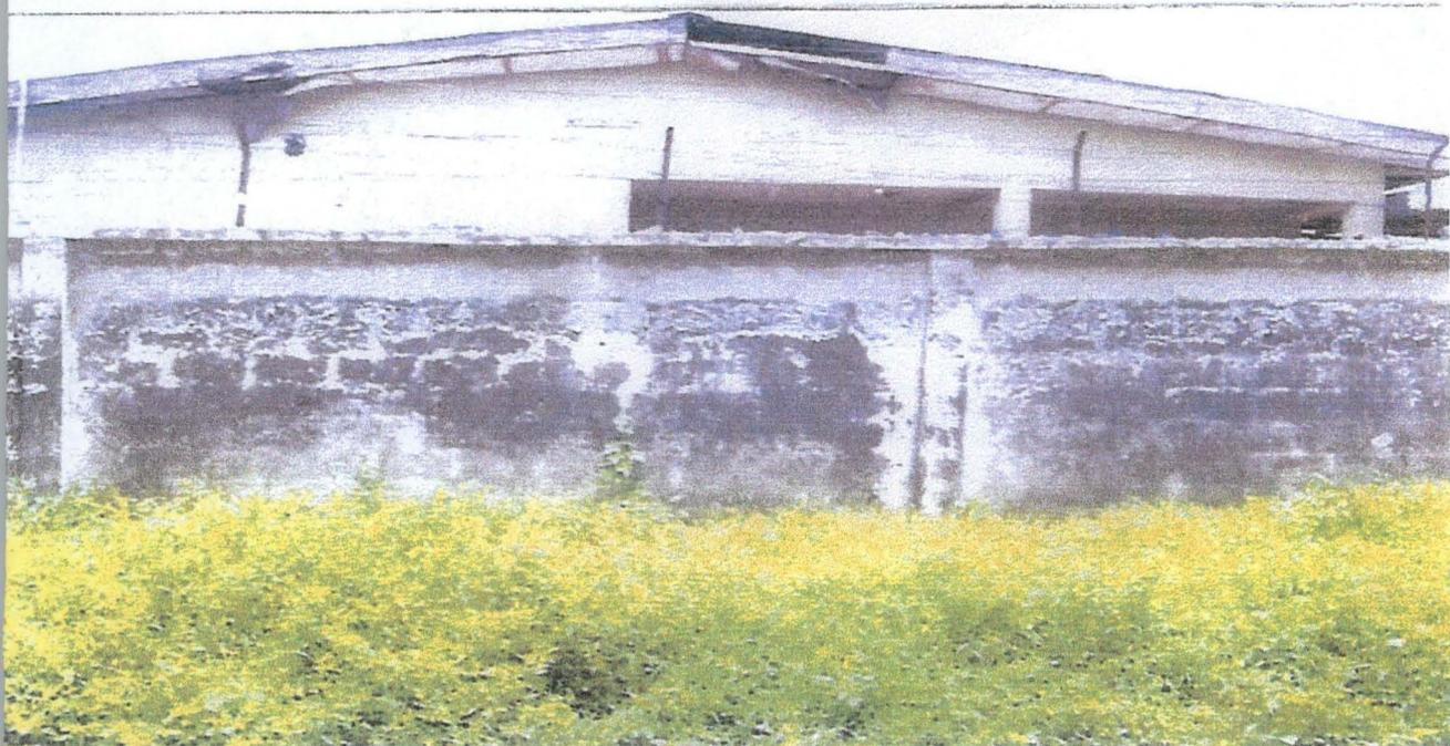
**Plate 2:** Shows the effect of rain on wall surface resulting to discoloured paint wall, rendering flaked exposing the blocks with part of fascia board and ceiling board decayed and falling off.
