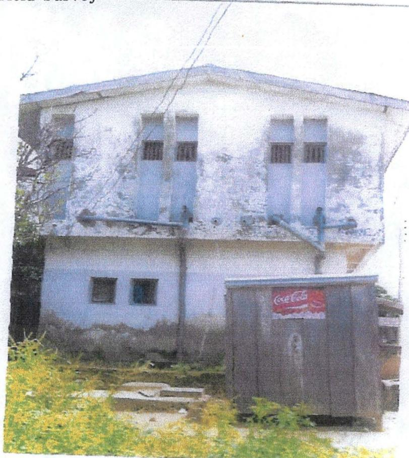
**Plate 10:** Shows a storey building affected by rainstorm causing discolouration of the wall at the first floor of the building and underground moisture at the ground floor in Chanchaga town.
