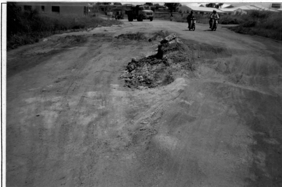
Plate 6 Roughness and lack of camber on paved road.
