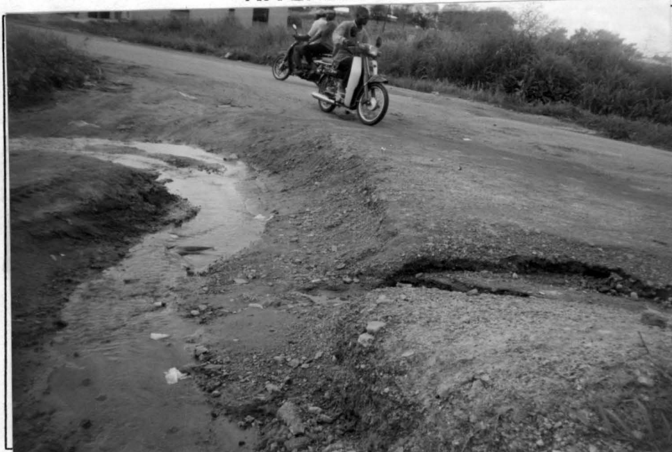
Plate 4 Standing water and pothole on paved road.
