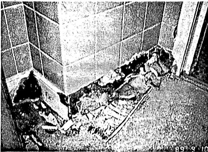
**Plate 3.2 Rotting of timber skirting caused by rising damp**
