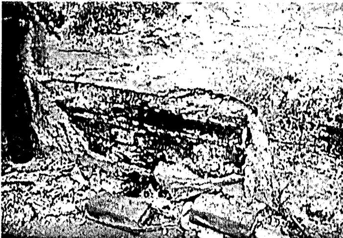
**Plate 3.3 Wall damaged by rising damp**
