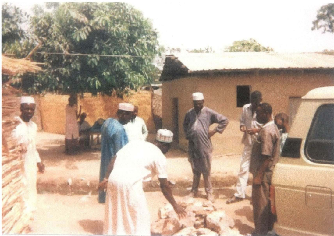
Plate xiv: Arranging rocks to build a solar dryer in a fisherman's compound
