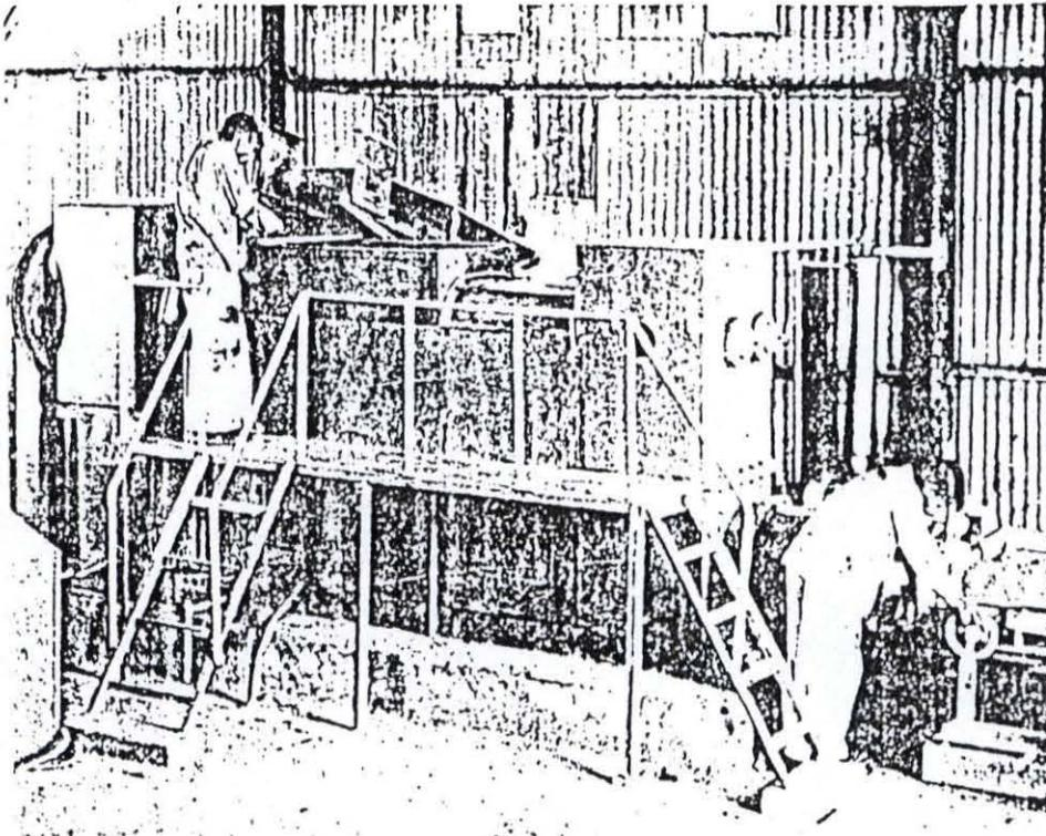
FIG. 4ii SEMI-MECHANISED BRICK MACHINE
