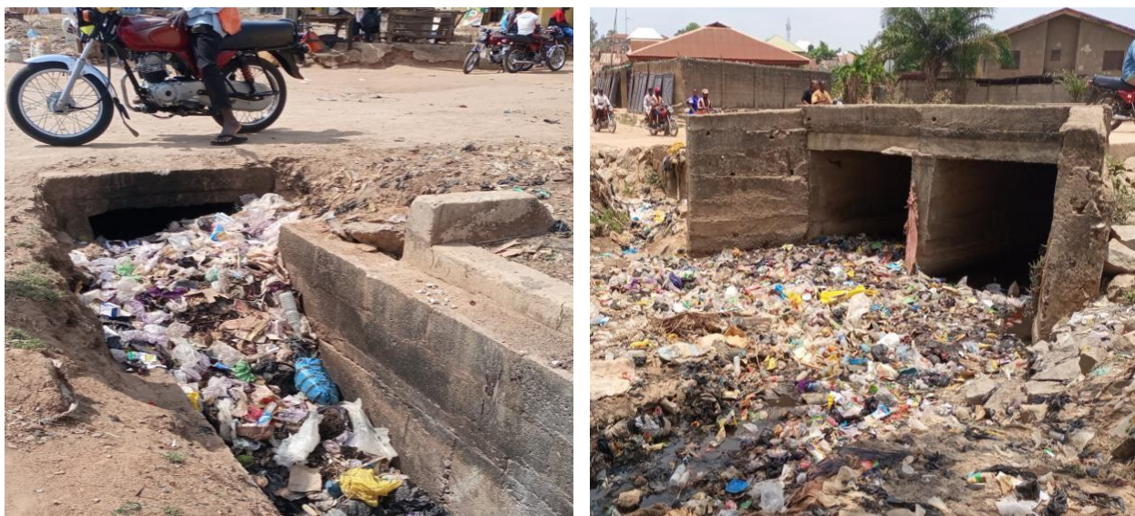
Plate II: Blockage of drainage and water ways due to improper waste disposed Source: Author's Field Survey, 2021
