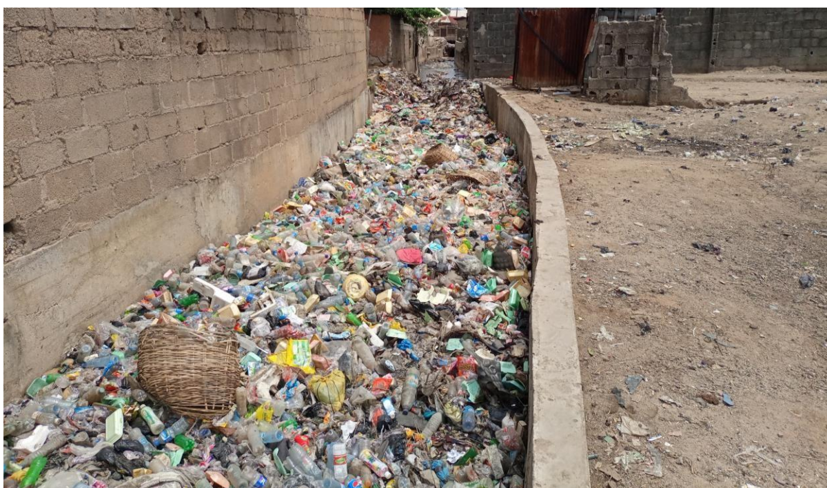
Plate III: Drainage blocked by waste in Bagama, Suleja – Main cause of urban floods
