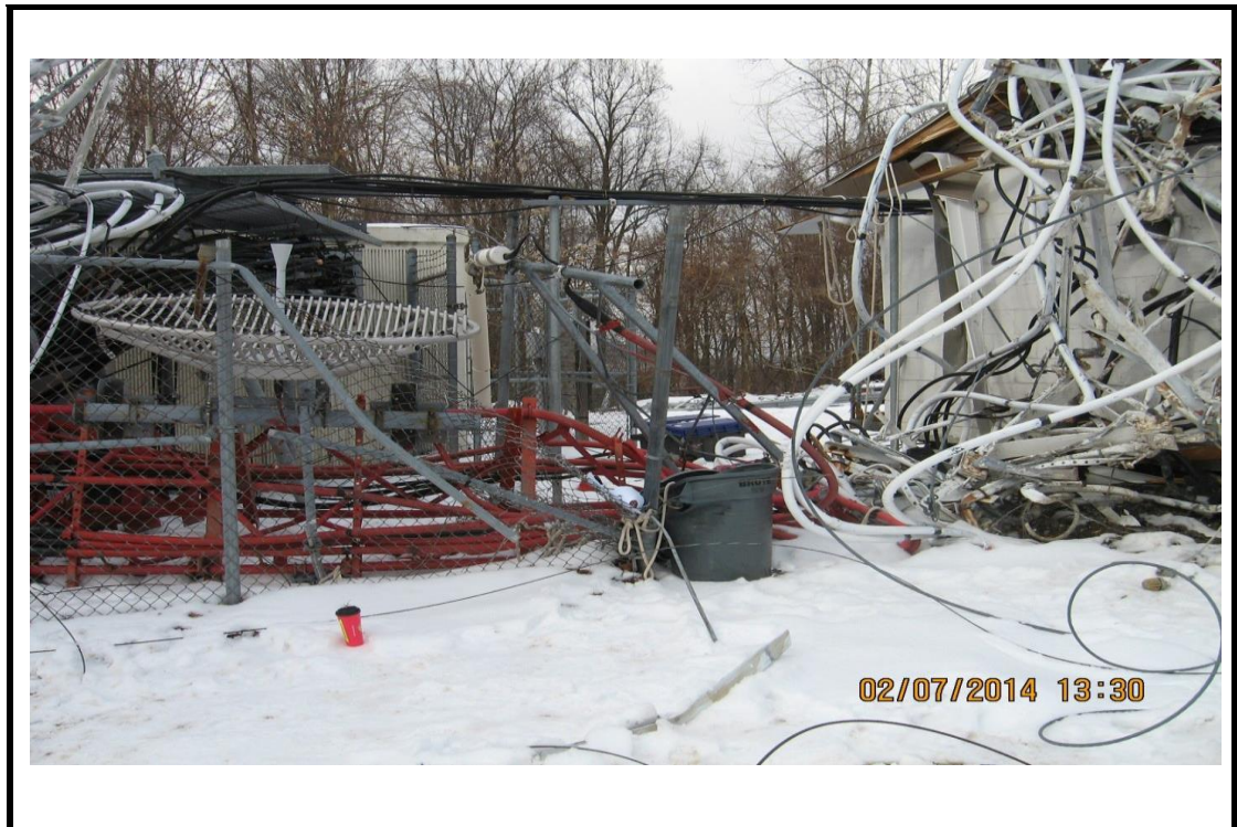
Plate III: Collapse of a Telecommunication Tower at the Summit Park Community in Clarksburg, Wv (Muhammad and Scott , 2014 a)
