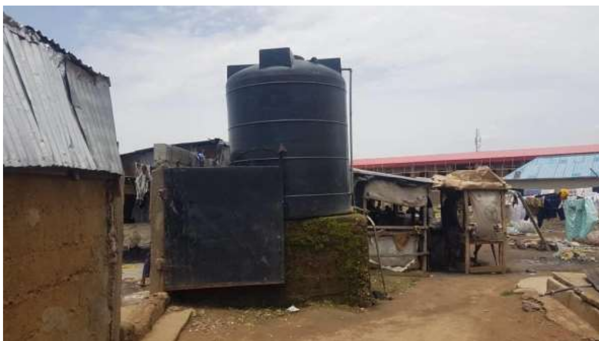
Plate 10: Typical Water Tank for a Commercial Borehole Source: Author's Field Survey, 2021
