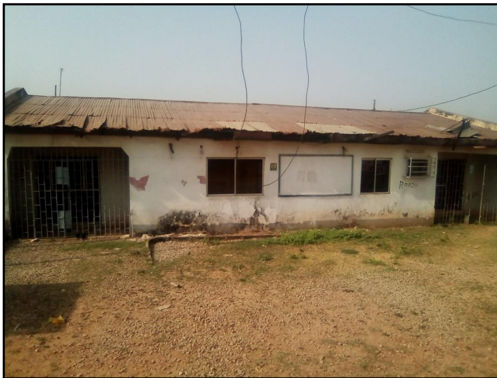
Plate I: A Vacant Buildings with Loose Roof Parts in Phase III Residential
