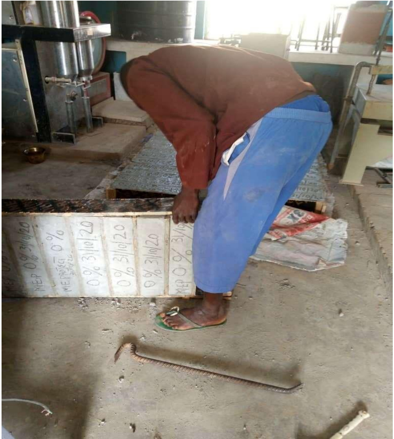
Plate XIX: Removal of formwork from the concrete beam
