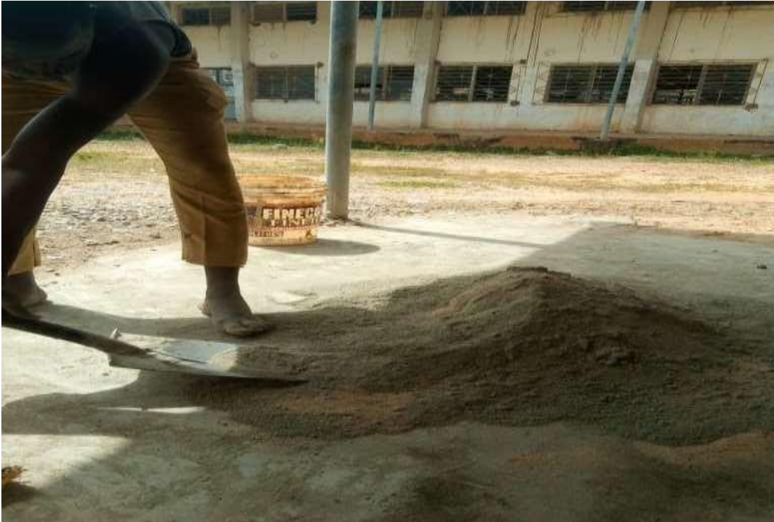
Plate XI: Mixing of concrete at Federal Poly Bida Civi1 Engineering Laboratory
