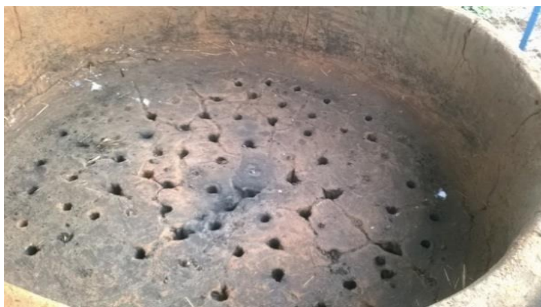
Plate VIII: Internal Perforation of the Traditional Oven (Saba et al. , 2017)
