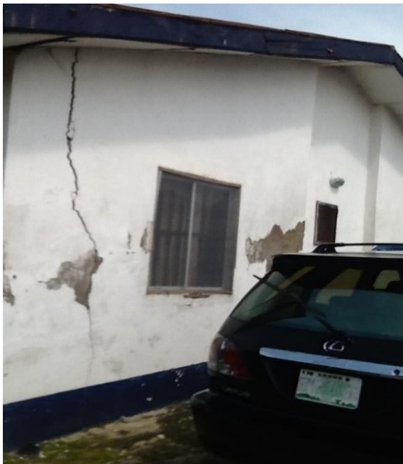
Plate I: Cracked wall at Phase IV
