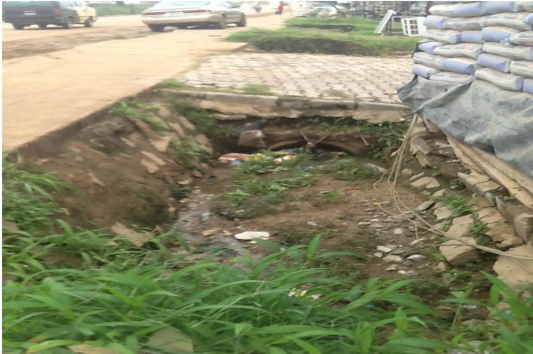
Plate VIII: Blocked drainage along Byazhin road
