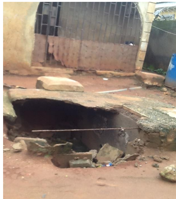
Plate X: Dilapidated septic tank at Byazhin Source: Field survey, 2019
