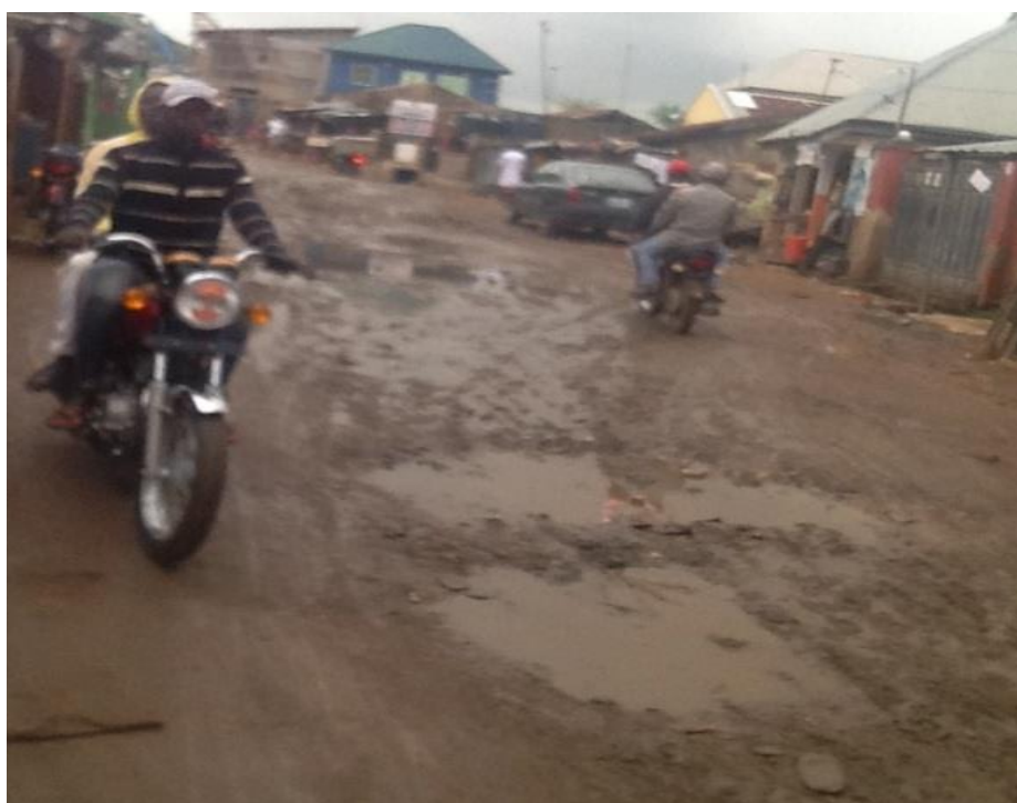
Plate VII: Access road without drainage at Byazhin
