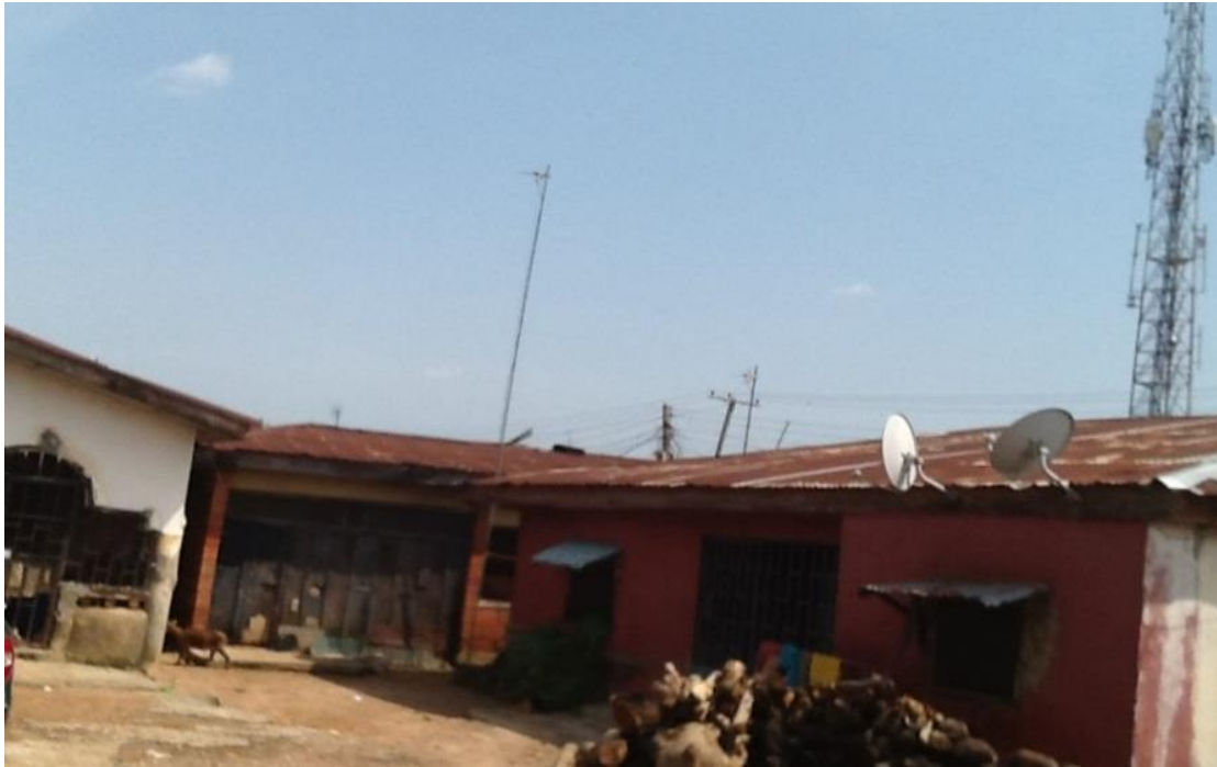
Plate III: Rusting and leaking roofing sheet at Phase II side II
