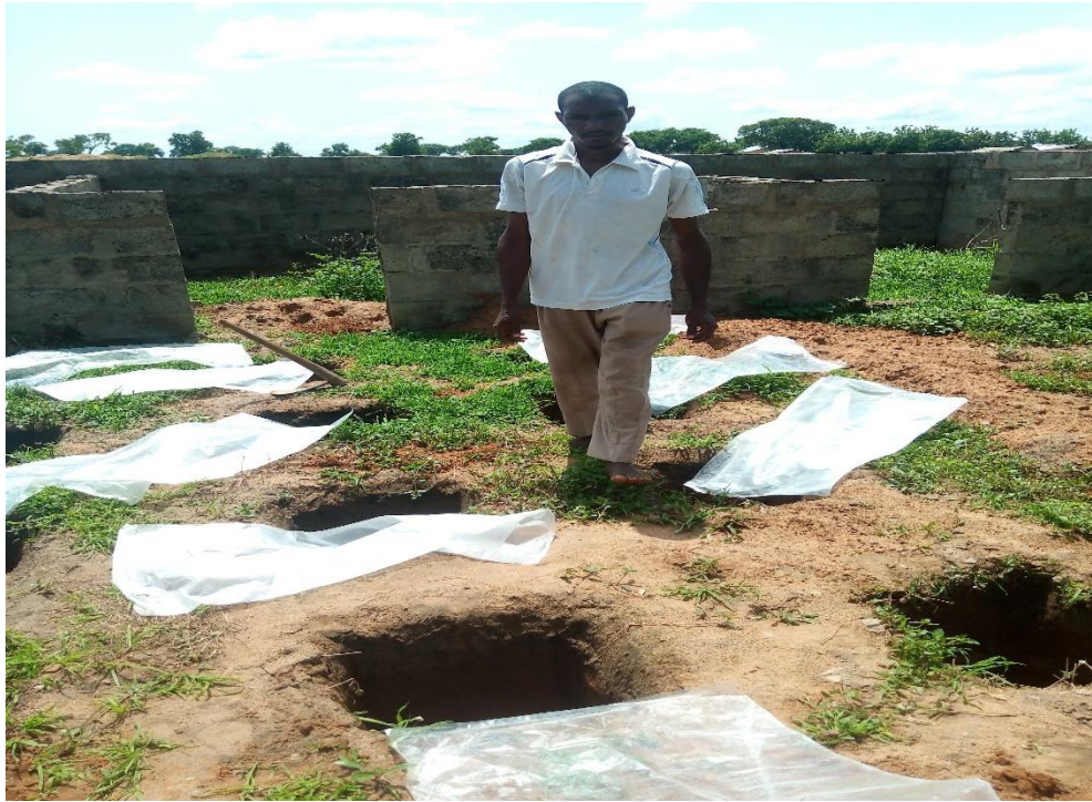
Plate IV: HDPE used to line the pits
