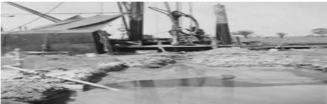
**Plate VI:** Unlined drilling fluid sumps were commonplace before the environmental consequences were recognized (Winter, 2017)
